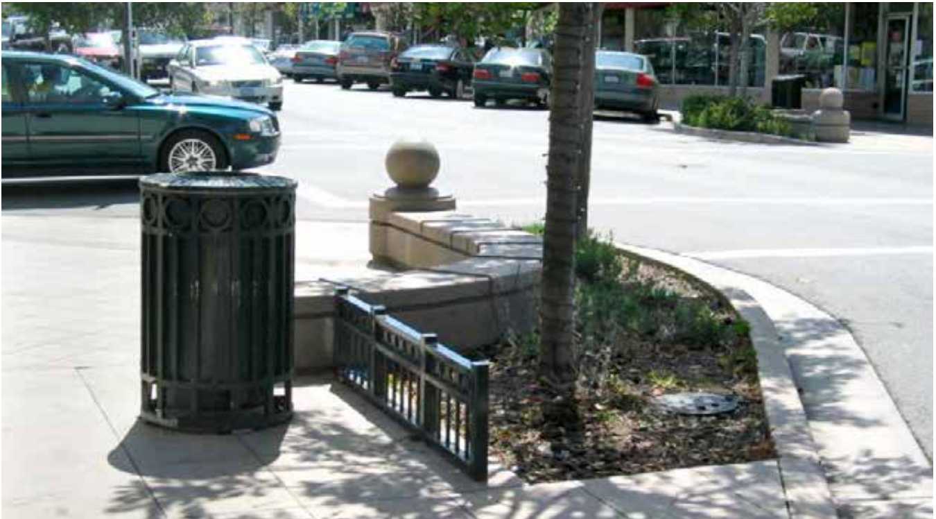
An example of a bulbout with tree planting and amenities in Burlingame, California.
