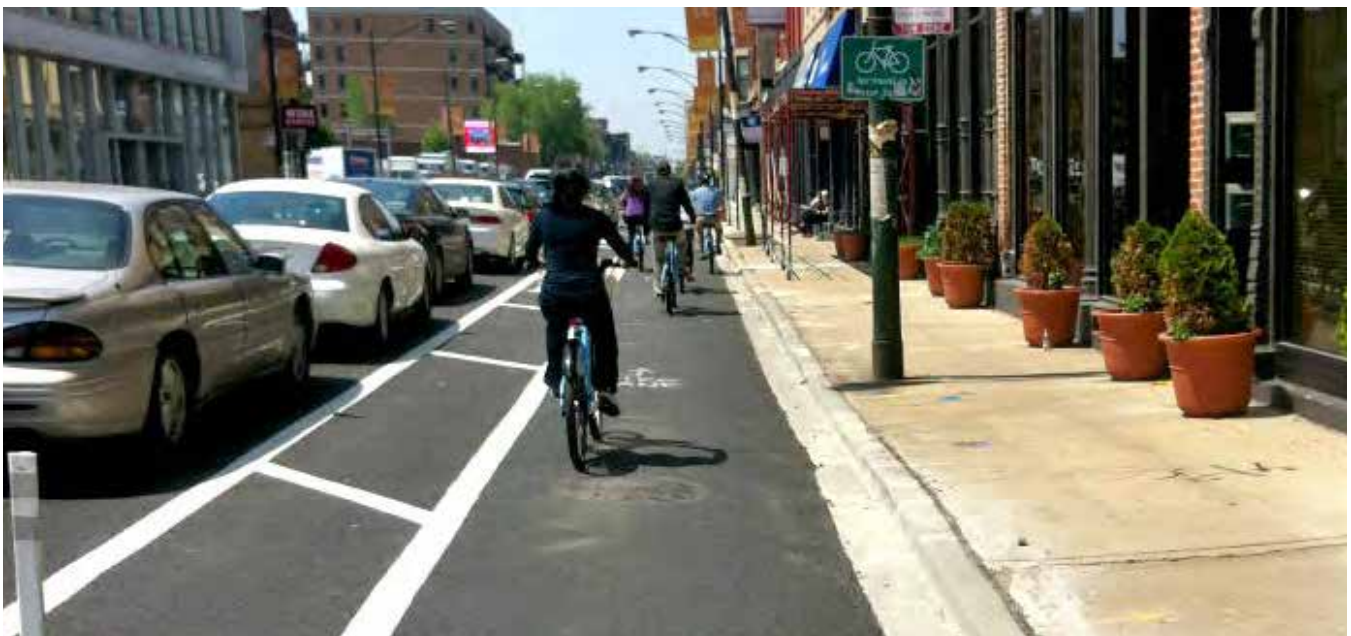
An example of a parking lane and buffer between bicycle lane and travel lane in St. Louis, Missouri.
