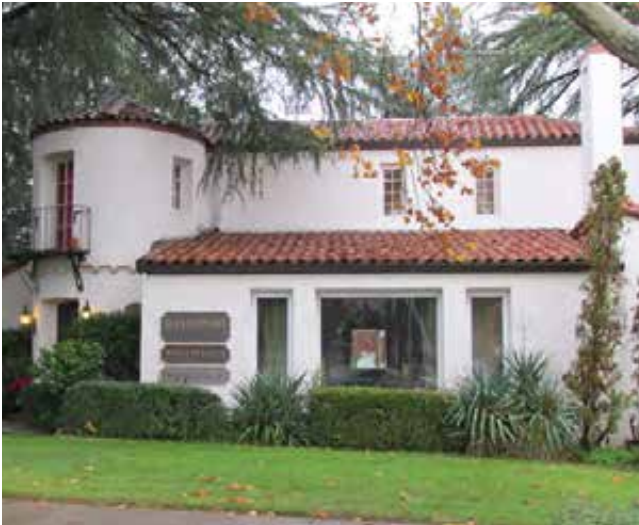
Downtown Redding has a range of office uses in a range of building types.
