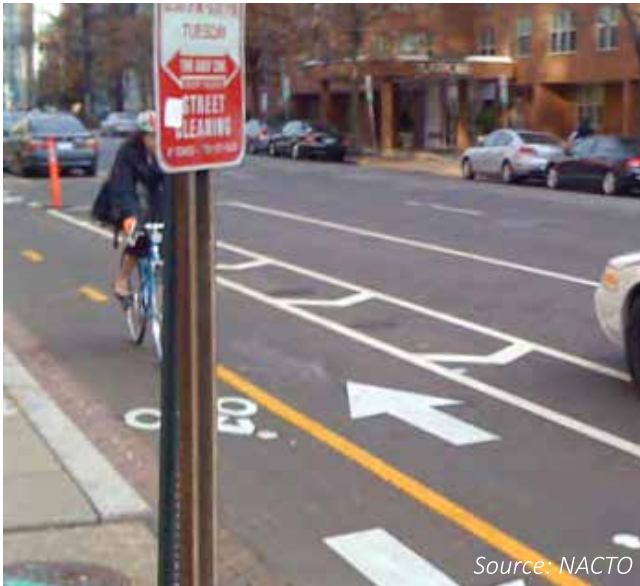
An example of a protected two-way bicycle track in Washington DC.
