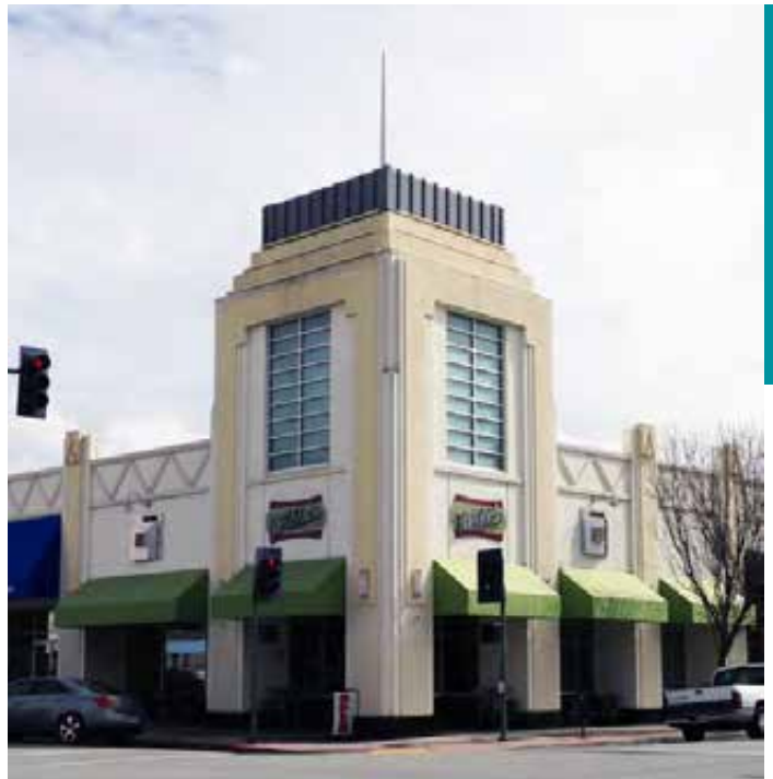
Along with the historic red brick buildings, art deco buildings characterize Downtown today.
