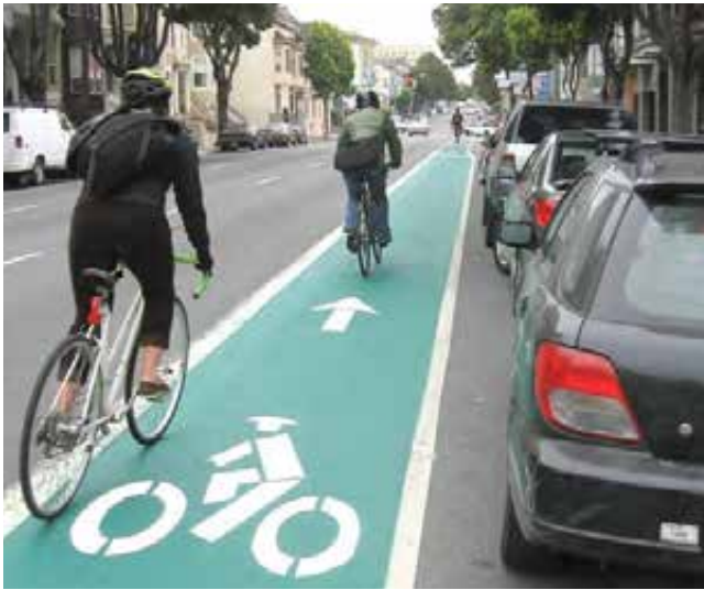
An example of a painted bicycle lane next to a parking lane.
