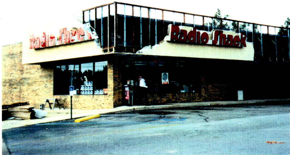
Figure 4-7. Building Facade Damaged -- Clearview, Florida
