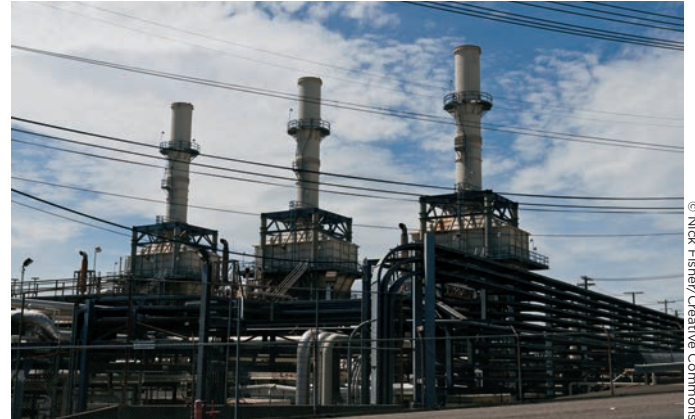
Part of the Chevron refinery in Richmond, CA.
