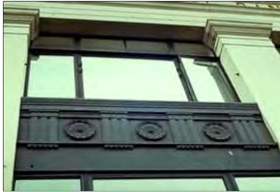
Historic steel sash can be fitted with dual glazing to improve thermal efficiency. Photo: NPS files.
