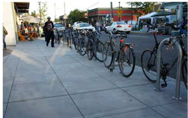
Standard staple or U-racks on a commercial street are aligned to provide clear path for pedestrians. Image from Nelson\Nygaard
