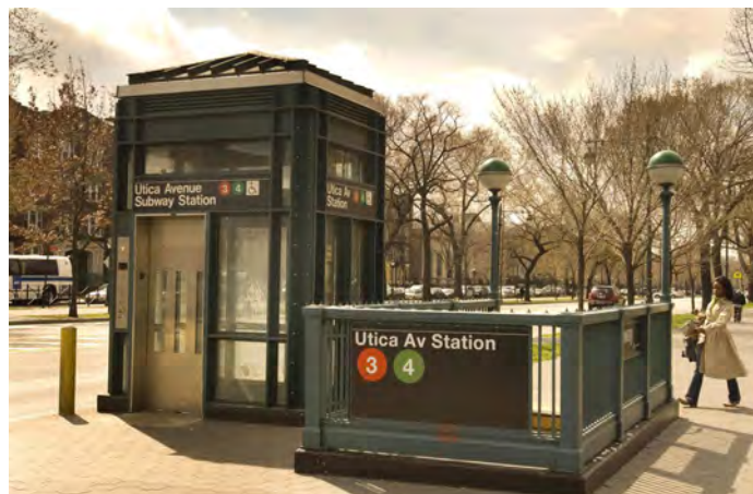
Accessible Elevator (New York MTA Utica Subway Station). Image from Nelson\Nygaard
