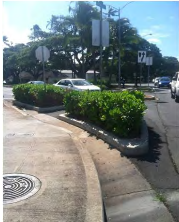
Planters are used to narrow the travel lane and create a tighter corner radius for vehicles (Honolulu, HI). Image from Nelson\Nygaard
