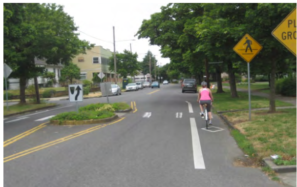
Mid-block crossing and “choker” island helps to reduce vehicle speeds (Portland, Oregon). Image from Nelson\Nygaard
