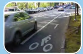
Dedicated bicycle facilities (bike lanes)
