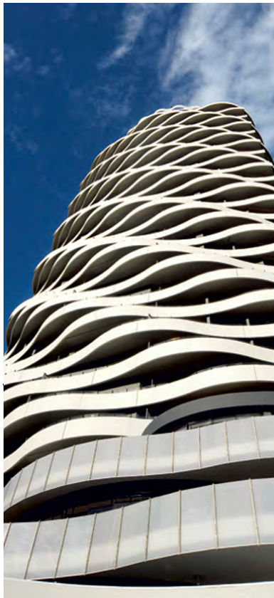
The Wave on the Gold Coast of Australia. The facade is made up of a lanai allowing each resident habitable outdoor space, views and shaded interior walls. Image from DBI Design
