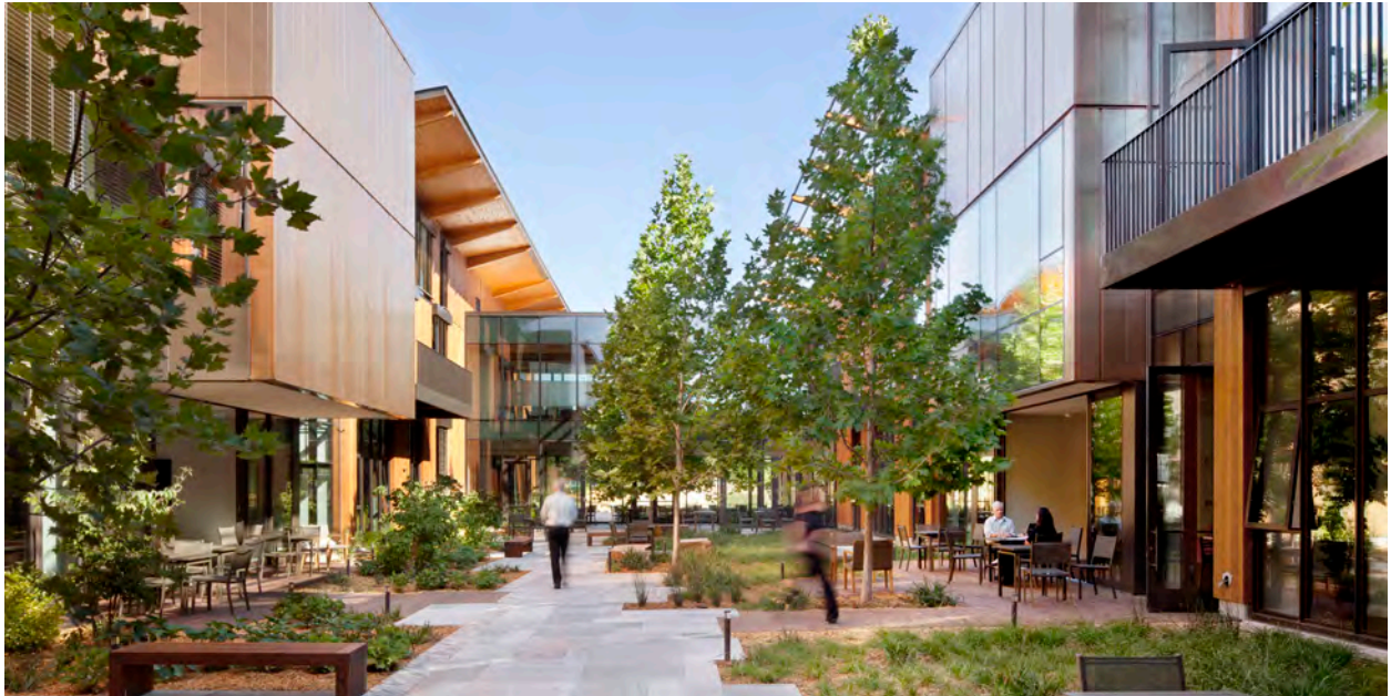
Packard Foundation in Los Altos, CA offices include a courtyard for socializing, and access to light and air. To reduce energy use, the building's offices are daylit with skylights and clerestories. Image from Jeremy Bitterman, EHDD Architecture
