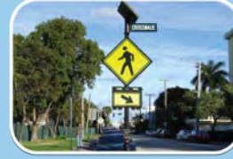
Rapid flashing beacons
