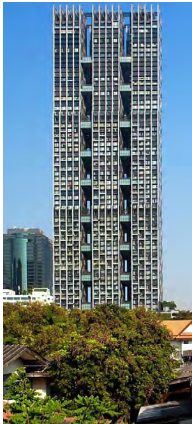
The Met Tower, Bangkok incorporates outdoor spaces, balconies and sky gardens. In this project, cross ventilation is used to cool and ventilate the apartments. Communal spaces are included on multiple stories. Image from WOHA designs
