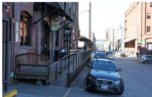
The shared street that evolved through the development of an older warehouse district in NW Portland became a favorite of locals, so much so, that the street character was replicated for new development fronting the street. These photos show a historic area in the neighborhood and more recent development.
