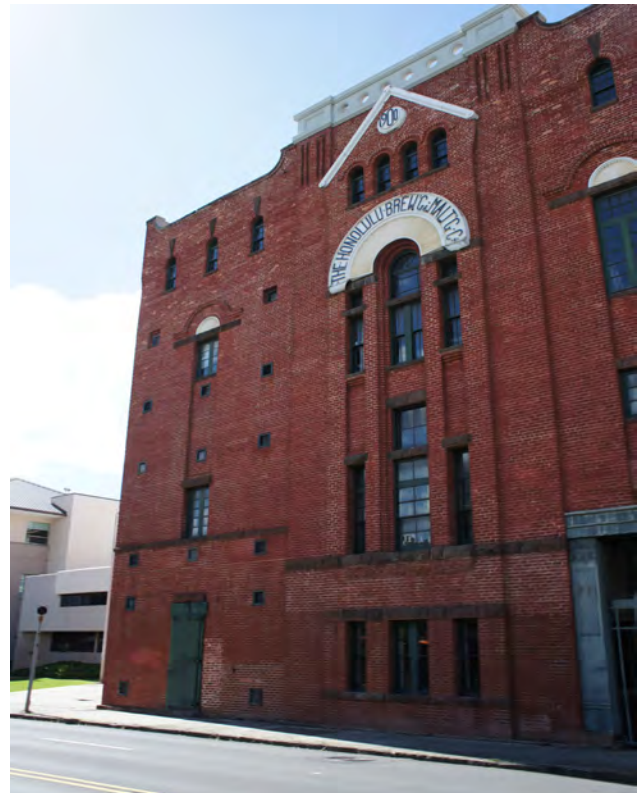
The Honolulu Brewery building on Queen Street is one of the few historic buildings surviving in Kaka`ako from the City's streetcar days. Image from Nelson\Nygaard
