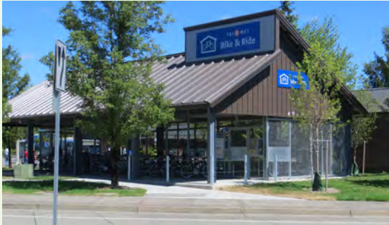
A card-access bicycle parking facility at a suburban TriMet light rail station. Image from Nelson\Nygaard
