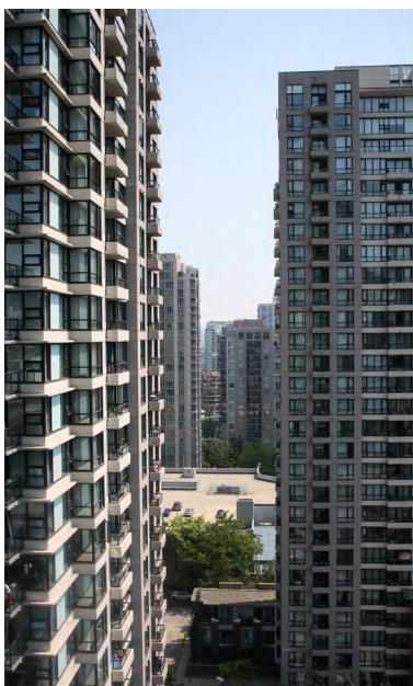
City of Vancouver 80' tower spacing required between residential projects (less for commercial projects). Image from VIA Architecture.
