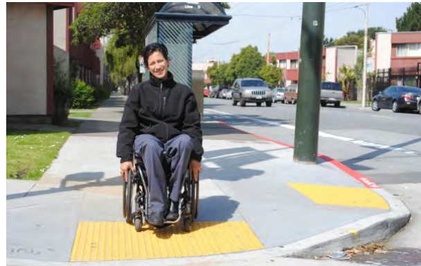
Accessible curb ramp. Image from San Francisco Department of Public Works.
