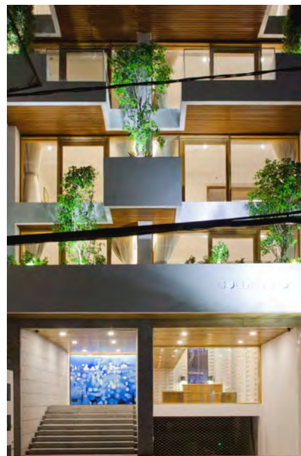
Golden Holiday Hotel, Vietnam's facade was designed to take advantage of the tropical weather with internal atrium, cross ventilation planted balconies with trees averaging 10' high. Image: Hiroyuki Oki Architectural Record Viet A Architects
