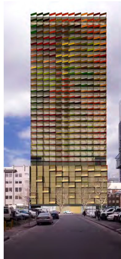
The Beckett Tower has a brightly colored facade with lanai acting both as shading and decorative device. Image from Elen Fraser Architecture
