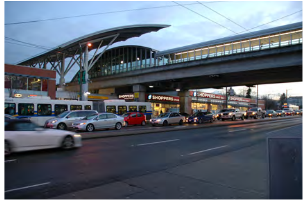
Broadway Commercial Skytrain Station Hub, Vancouver BC Image: VIA Architecture
