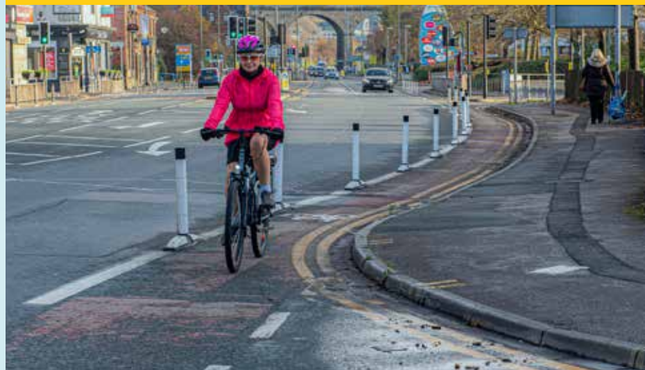
▼ Wand orcas have been implemented in several locations in the city during the pandemic as a quick way to provide segregation between cyclists and motorists.
