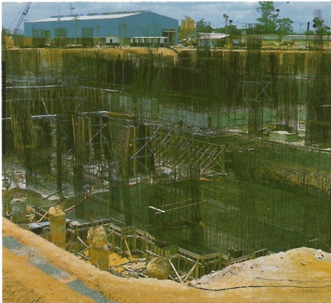
Top: Alcan's Greensboro, Georgia plant, which will have a new sheet ingot casting center, recycles used beverage cans and other aluminum scrap.
