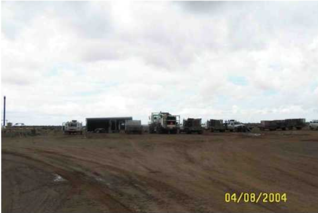
Figure 3-6. Equipment staging for 3D9C acquisition
