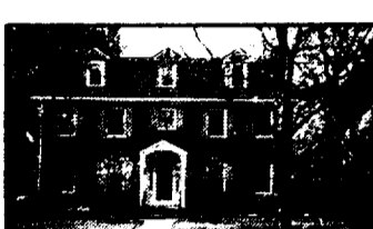
MOROSS ROAD Classic Williamsburg Colonial. Family Room. Walk to Pier. $550,000
