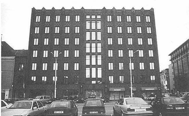
The front of the Tallinn City Government building, an outstanding example of Art Deco, changed into an expressionless face when PVC units were installed in 1994.
