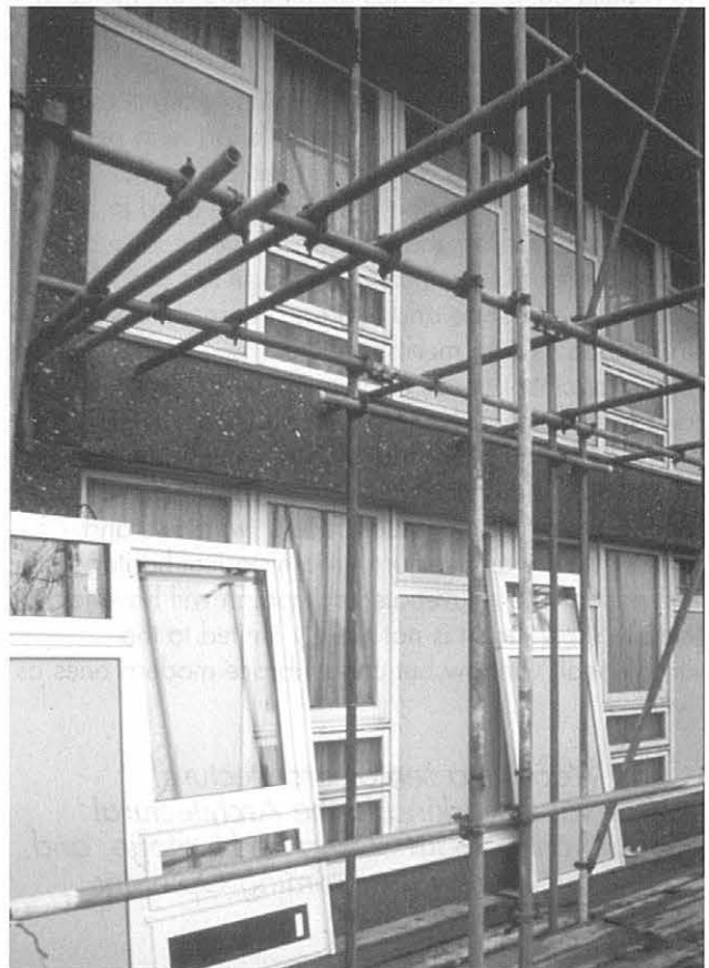
Original timber double glazed windows in situ shown against proposed PVC replacements which were rejected at Balfron Tower, East London.
