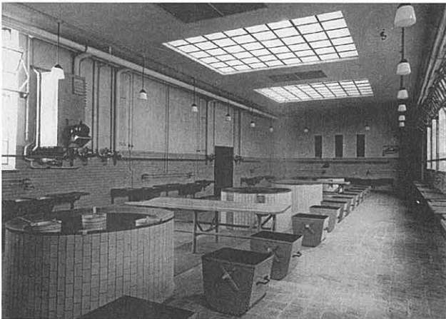
The windows of the Helsinki Abattoir production facilities opened simultaneously by operating a horizontal bar. Period photo: PeKo archives.
