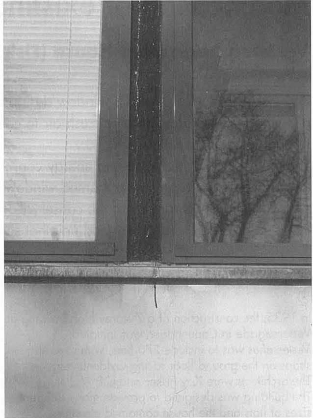
New detail at separation wall.
