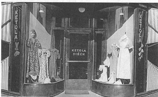
Corner entrance of a 1930s commercial building in Tampere with rounded steel windows, probably assembled from imported profiles at the Pietarsaari machine workshop. Period photo: Pietarsaari City Museum, PeKo archives.
