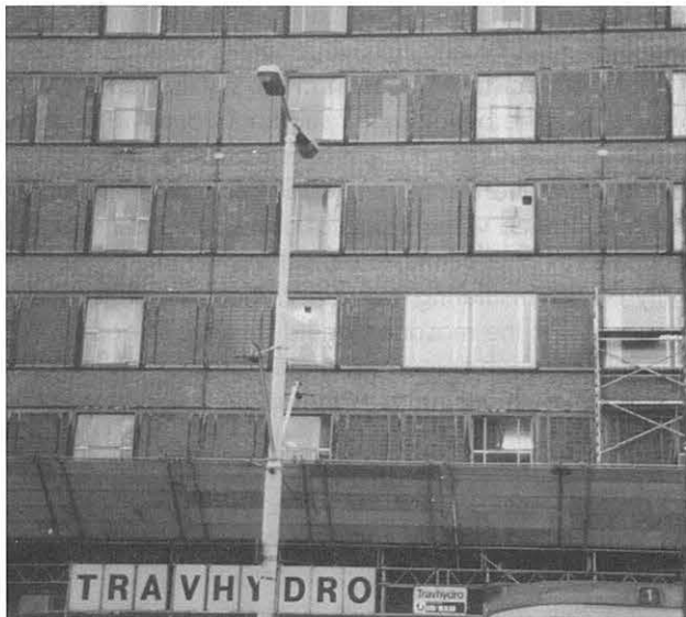
Full-size mock-up to test the aluminium replacement windows.
