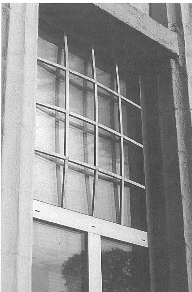
PVC windows aesthetically compromise this 1912 traditional building in Tallinn's Koidula street.
