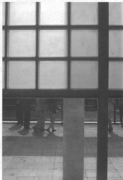
Transparent and translucent parts of the restored facade. Photo: Ola Wedebunn.
