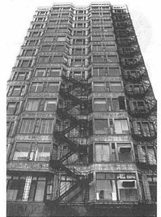
North facade before restoration, 1994. Photo: T. Gunny Harboe.
