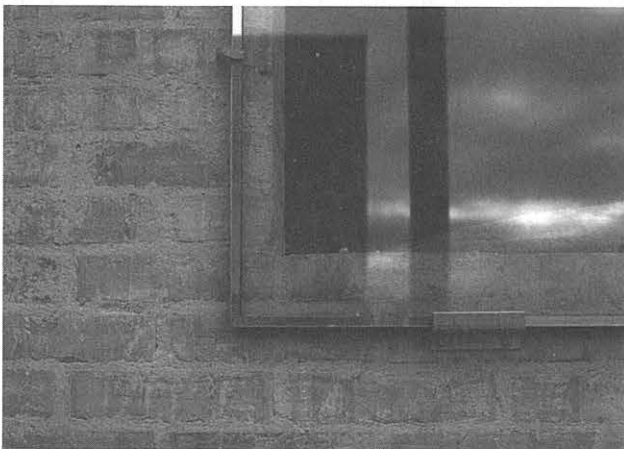
Double glazing unit at Tinggården, similar to technique used by S. Lewerentz. Photo: Peter Sørensen.
