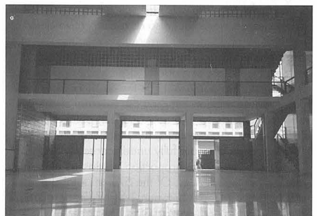
The poor daylight quality in the central atrium before restoration. Photo: Wessel de Jonge.
