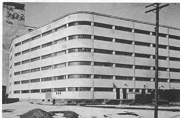
The SOK cooperative warehouse in Viipuri, designed by Erkki Huttunen (1932) featured steel windows. Period photo: PeKo archives.
