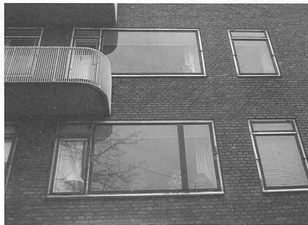
The rejected proposal for a division of the large window into two smaller units. Photo: Ola Wedebrunn.
