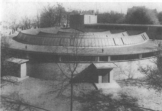
Former employment centre by Walter Gropius in Dessau in 1928, with a view of the round building with the row of top lights in the exterior walls and the curved roof sheds.
