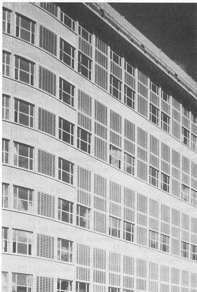
Detail of the restored facade showing the additional windows.
