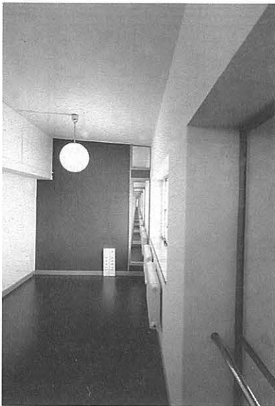
Where the partition meets the facade, a strip of glass allows to appreciate the original structure, to spread light between rooms and to keep sight lines. Photo: Mats Håkansson.
