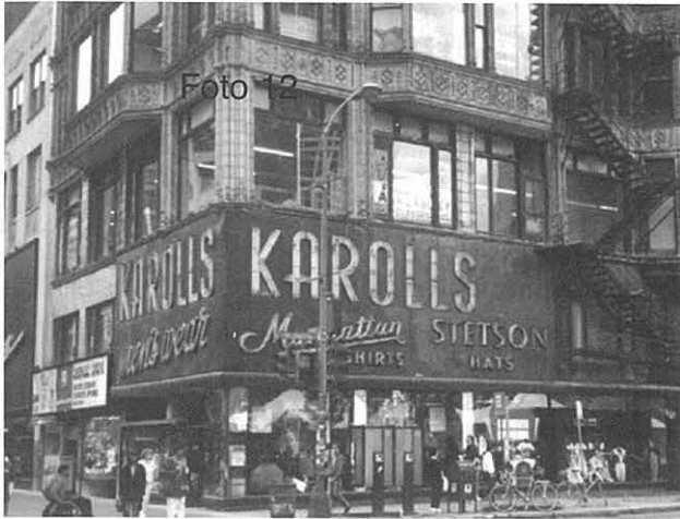
Store front before restoration, 1994. Photo: T. Gunny Harboe.
