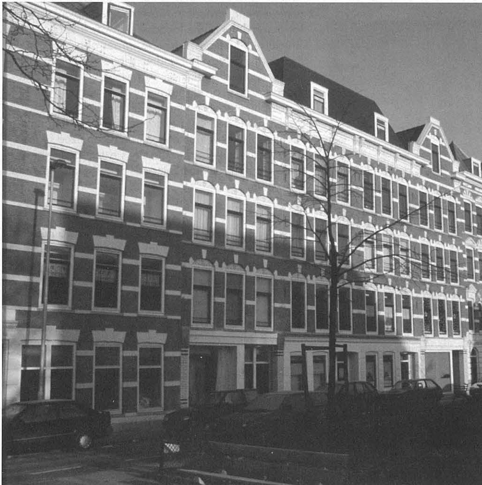
Typical 1900-1920s ring housing in Rotterdam after careful renovation. All illustrations by W. de Jonge except where stated otherwise.
