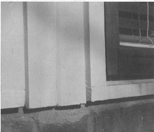
Detail of the replaced window casements with restored teak wood pivot windows. Photo: Thomas Tägil, 1999.
