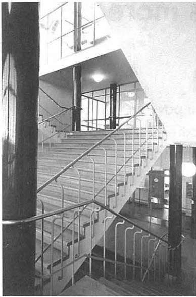
Many efforts were put in avoiding fireproof walls in the open staircase hall. Photo: Mats Håkansson.
