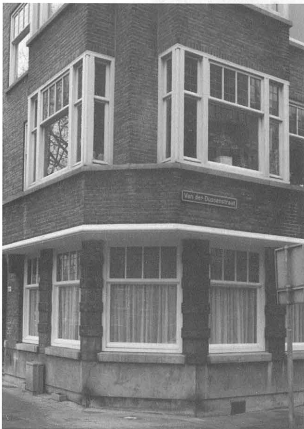
Typical 1920-1940s housing in Blijdorp, featuring horizontal timber windows with quite bold details.
