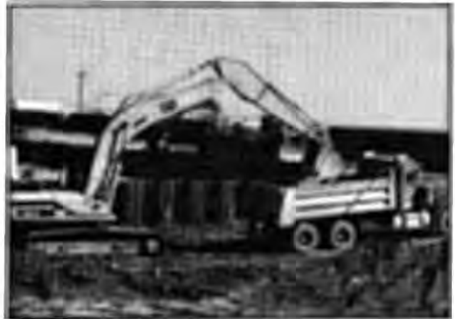
An excavator loads soil in a dump truck
