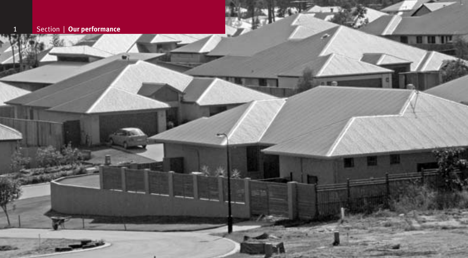
Planning for Varsity Station Village applied the principles of transit oriented development to create a master planned community
