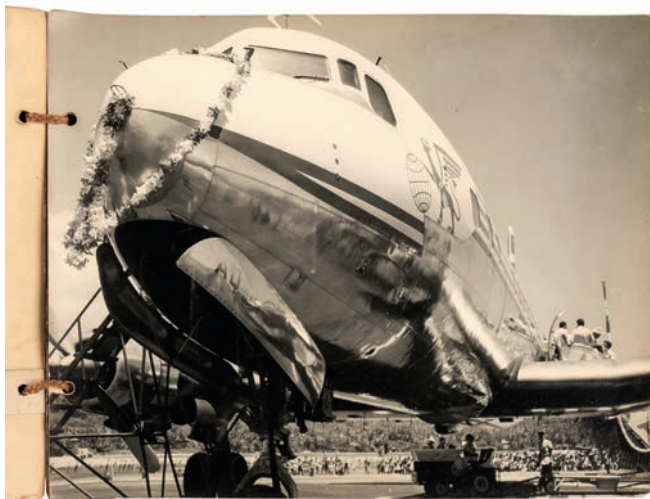
579* Tahiti Airport. A group of 20 photographs relating to the construction and opening of Tahiti International Airport, c. 1960, vintage gelatin silver prints on thin card, the first image of a plan, the others showing aerial views, digging, construction and opening of the airport with aircraft and people, contemporary French presentation inscription dated December 1960 to upper wrapper, punch holes to left margins with string ties, a little edge wear, images 24 x 30cm (1) £100 - £150
