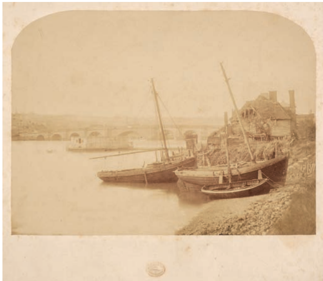
472* Archer (Frederick Scott, 1813-1857) . Rochester Bridge, c.1855, albumen print, arch top, 164 x 221mm, original thin card mount with photographer's embossed stamp to lower margin This photograph is taken from the castle and cathedral side of the bridge and features boats and a rustic timber building in the foreground. (1) £200 - £300
