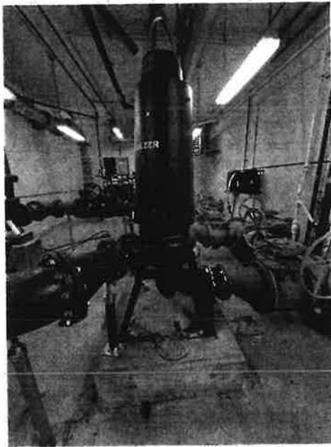
Figure 1. Pumps #2 and #3 installed at Niantic Pumping Station in East Lyme, CT. There are minor differences between each pump system, such as the flexible joint at the suction elbow.
