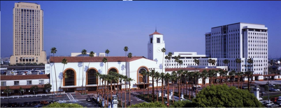
View from Alameda Street
