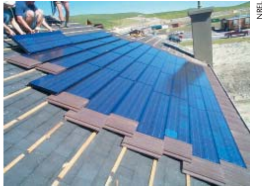
Solar PV roof tiles.
