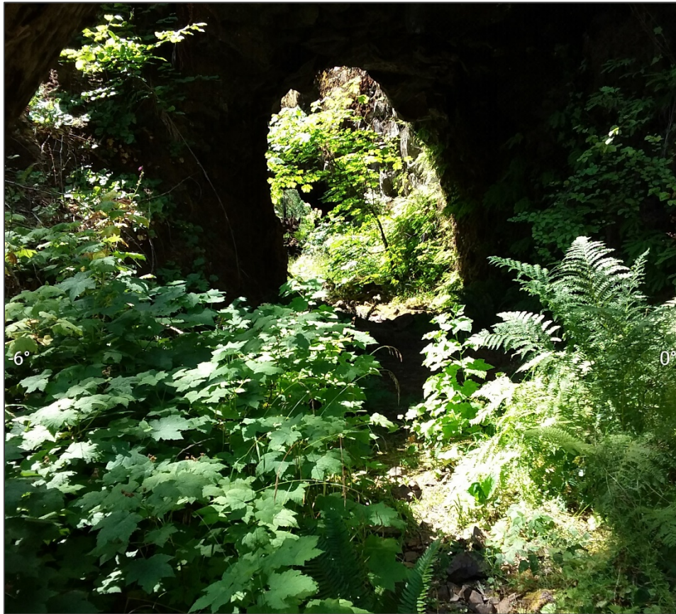
Figure 28. Tunnel leading to the lower falls along South Fork Clackamas River
