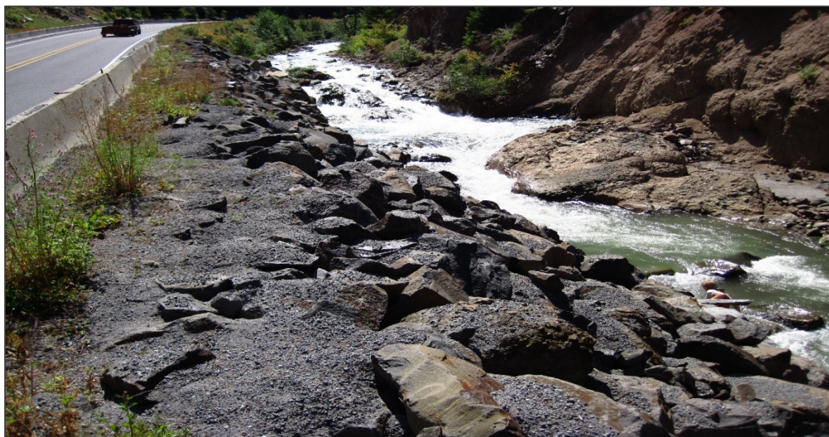
Figure 30. Highway 35 adjacent to East Fork Hood River
