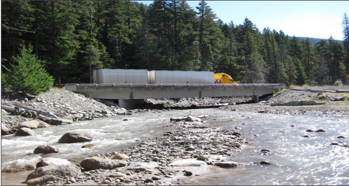
Figure 31. Polallie Bridge over East Fork Hood River
