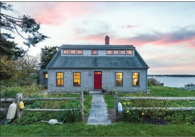
Originally built in 1938, this historic Cape has been expanded and renovated down to the studs.
