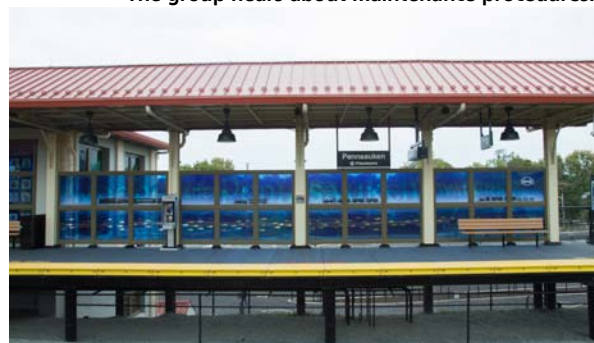
NJ Transit Atlantic City Line Pennsauken station.
