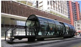
When faced with high ridership problems due to a conventional boarding systems, Lerner created revamped glass tube stations that enabled faster boarding through multiple doors, where passengers pay fares before entering the station. The new "tube stations" opened in October 1991 as part of the first Ligeirinho express line. Today there are 357 tube stations throughout the city.
