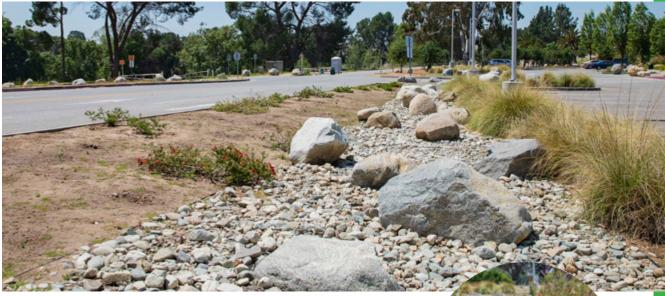
Left: Curb side infiltration trench between street and parking lot Right: Typical example of vegetation and boulders in an infiltration trench
