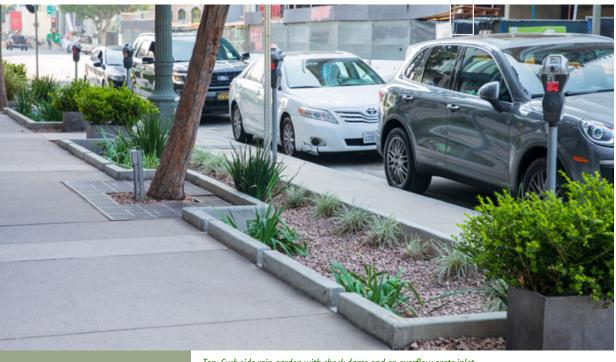
*Top: Curb side rain garden with check dams and an overflow grate inlet Bottom: Curb side rain garden with step out zone.*
