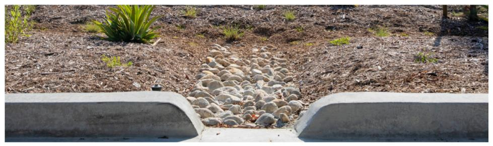
*Curb slot flow entrance with energy dissipator.*
