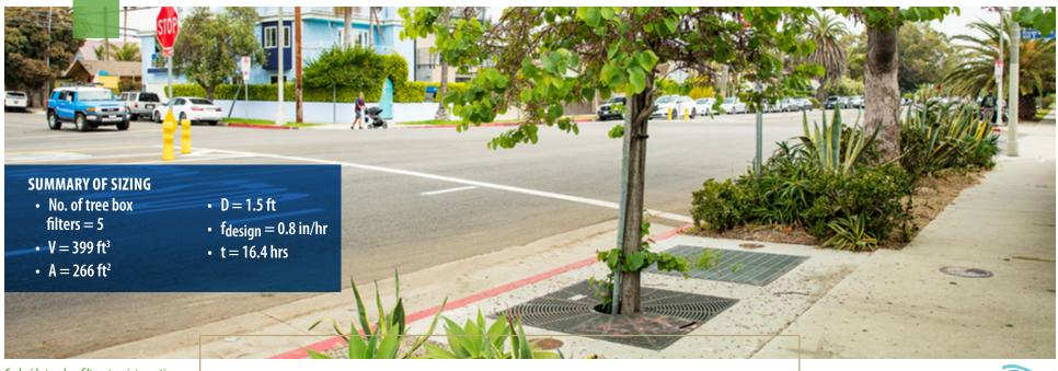
Curb side tree box filter at an intersection
