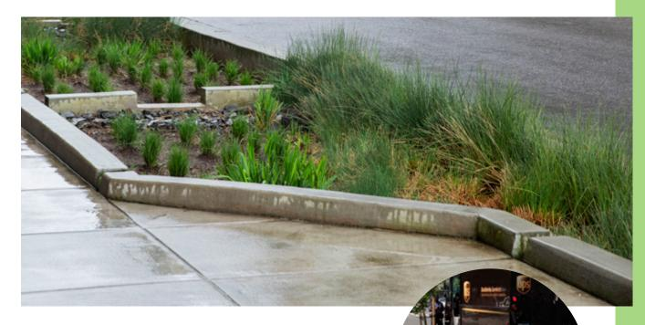
Rain gardens are vegetated areas depressed below the surrounding ground surface and surrounded by an impermeable barrier, such as a curb, with open slots that allow flow to enter. Water that enters the rain garden ponds up and slowly filters into the underlying soil, both reducing stormwater runoff volume and removing contaminants through physical and biological processes.
