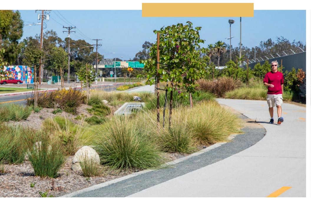
Curb side vegetated swale with meandering walking/biking trail
