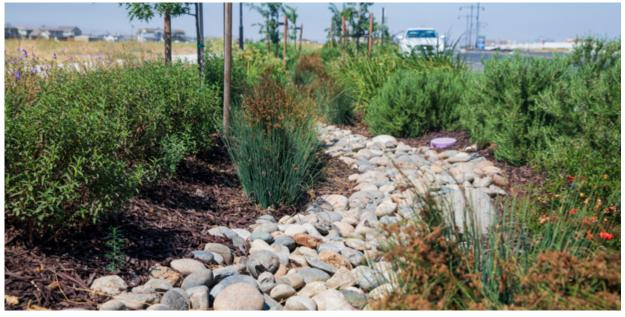
Median infiltration trench with vegetation lined edges.
