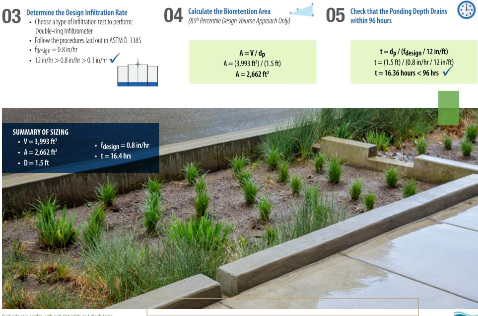
Curb side rain garden with curb slot inlets and check dams
