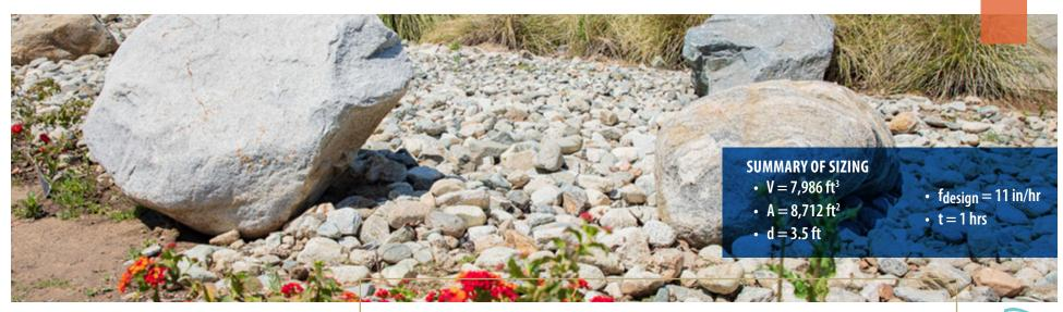
Curb side infiltration trench with varying rock sizes.
