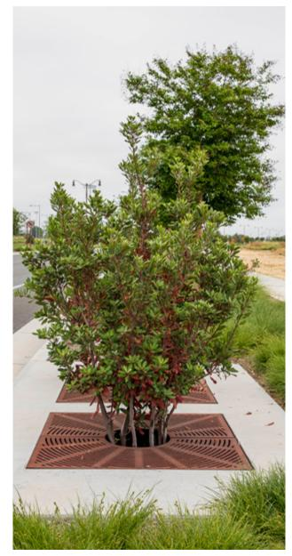
Curb side tree box filter placed in series.
