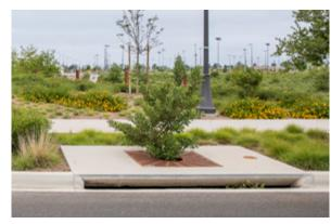
Curb side tree box filter separated from walkway.
