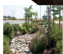
*Left: Curb side infiltration trench between sidewalk and building Right: Median infiltration trench with meandering flow line*
