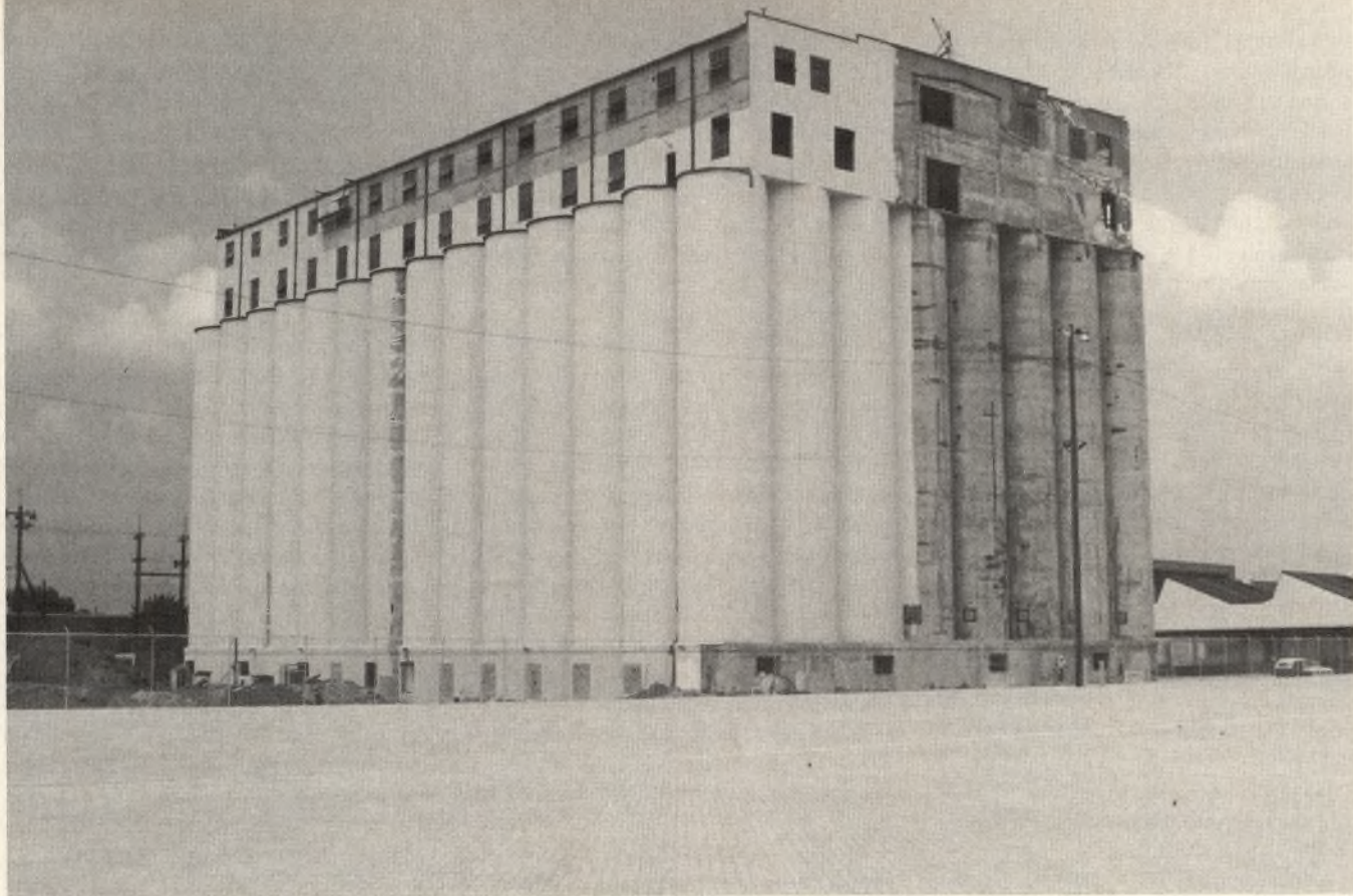
New Orleans' 72-year-old public grain elevator is being converted into a coffee silo and processing center.
