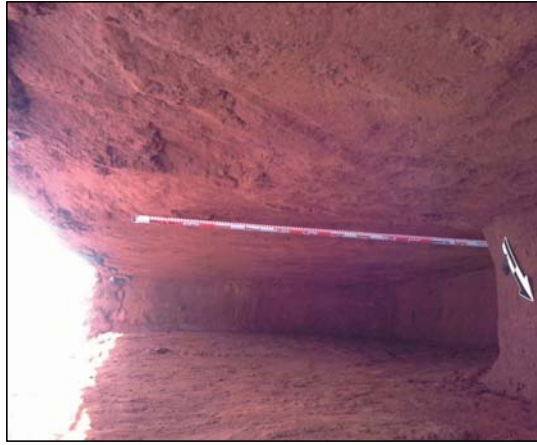
Figure 69. T-6, mid-trench view to southeast, noting mid-trench bench excavated for trench access and stability
