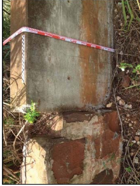
Figure 37. SIHP # -7758 Feature, contact between square-faced basalt boulders and concrete portions of the wall
