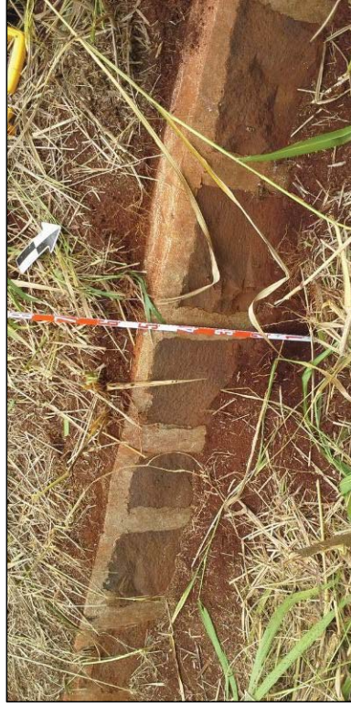
Figure 31. SIHP # -7758 Feature 2, irrigation ditch with square-faced basalt boulders, view to southeast
