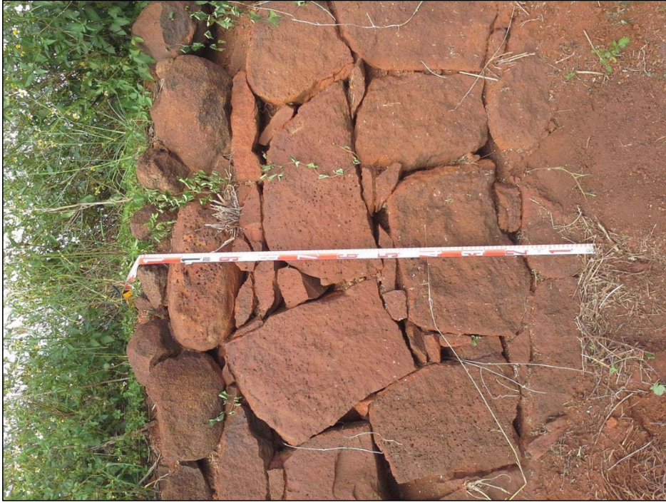
Figure 28. SIHP # -7758 Feature 1, road buttress and sediment trap, view to northwest
