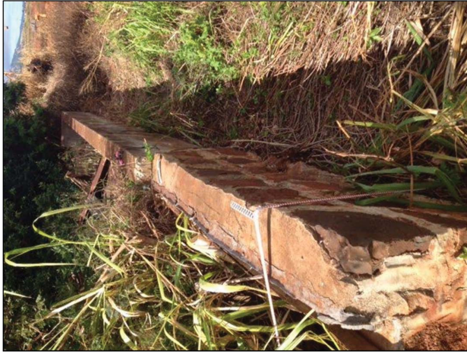
Figure 35. SIHP # -7758 Feature 4, general oblique view to northwest
