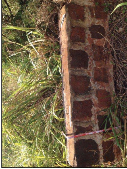
Figure 36. SIHP # -7758 Feature 4, square-faced basalt boulders and mortar portion of the wall
