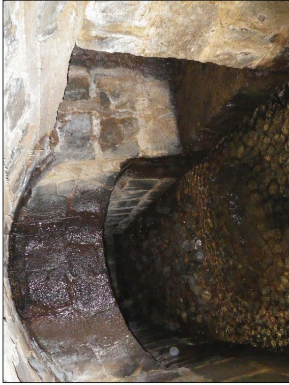
Figure 21. Inside the Kahana tunnel, upper Waiāhole Ditch, built 1929-1931 (Wai'anae Crider 2014)
