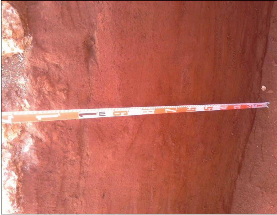
Figure 46. T-1, close up view of north west wall profile, noting lower boundary of Stratum I at approximately 1 m above base of excavation, view to north west
