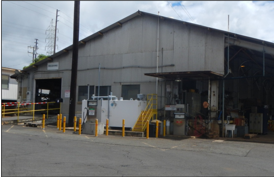
Figure 3.6 Photograph of Existing Fueling Area
