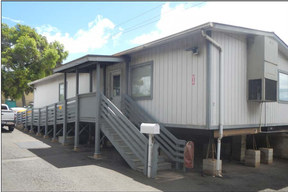
Figure 3.2 Existing C&M Office Trailer
