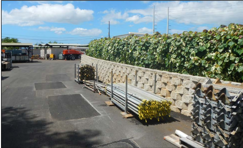
Figure 3.17 Improved Portion of Makai Former Wastewater Pond Berm
