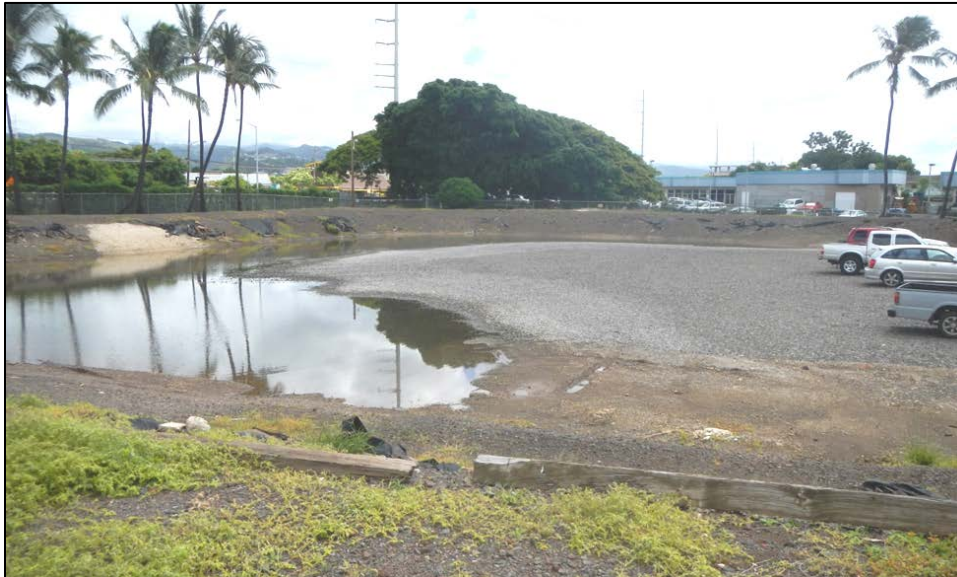
Figure 3.16 View from West Side of Mauka Former Wastewater Pond
