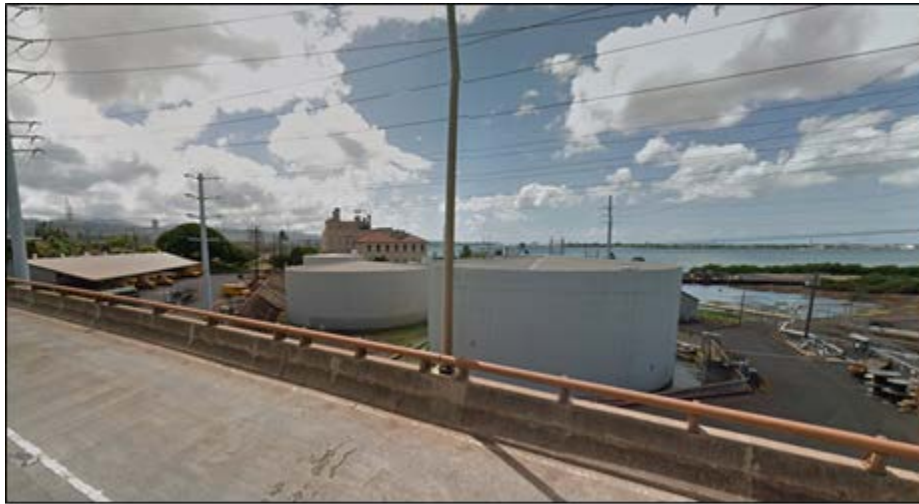
View southeast towards WGS from the makai lane of H-1 Freeway.
