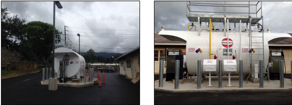
Figure 3.8 New Fueling Area at Ko‘olau Baseyard
