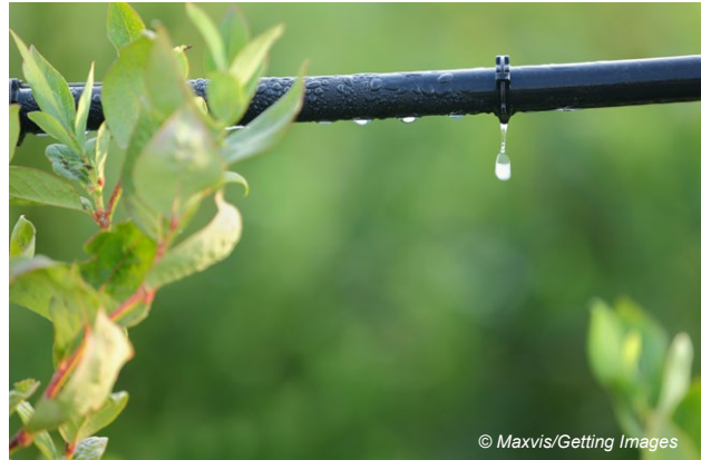
FIGURE 5 DRIP IRRIGATION SYSTEM IN GREENHOUSE
