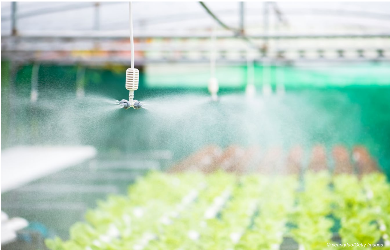
FIGURE 2 FOGGING TECHNIQUE FOR COOLING OF GREENHOUSES
