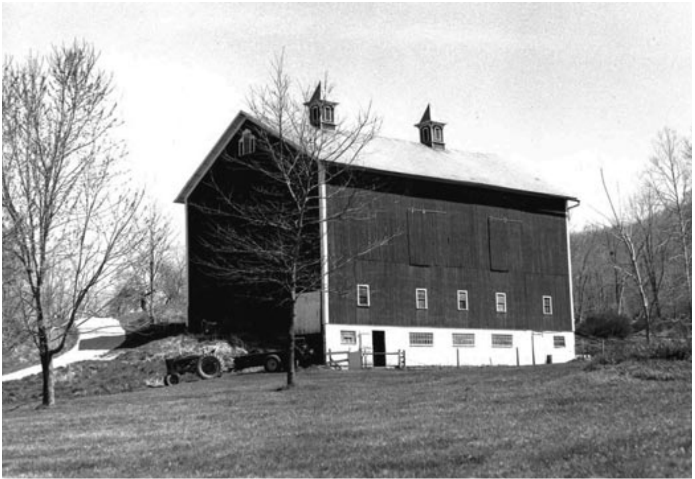
Above, at three stories tall, the Brown-Bender barn design was unusual for the Cuyahoga Valley area.
