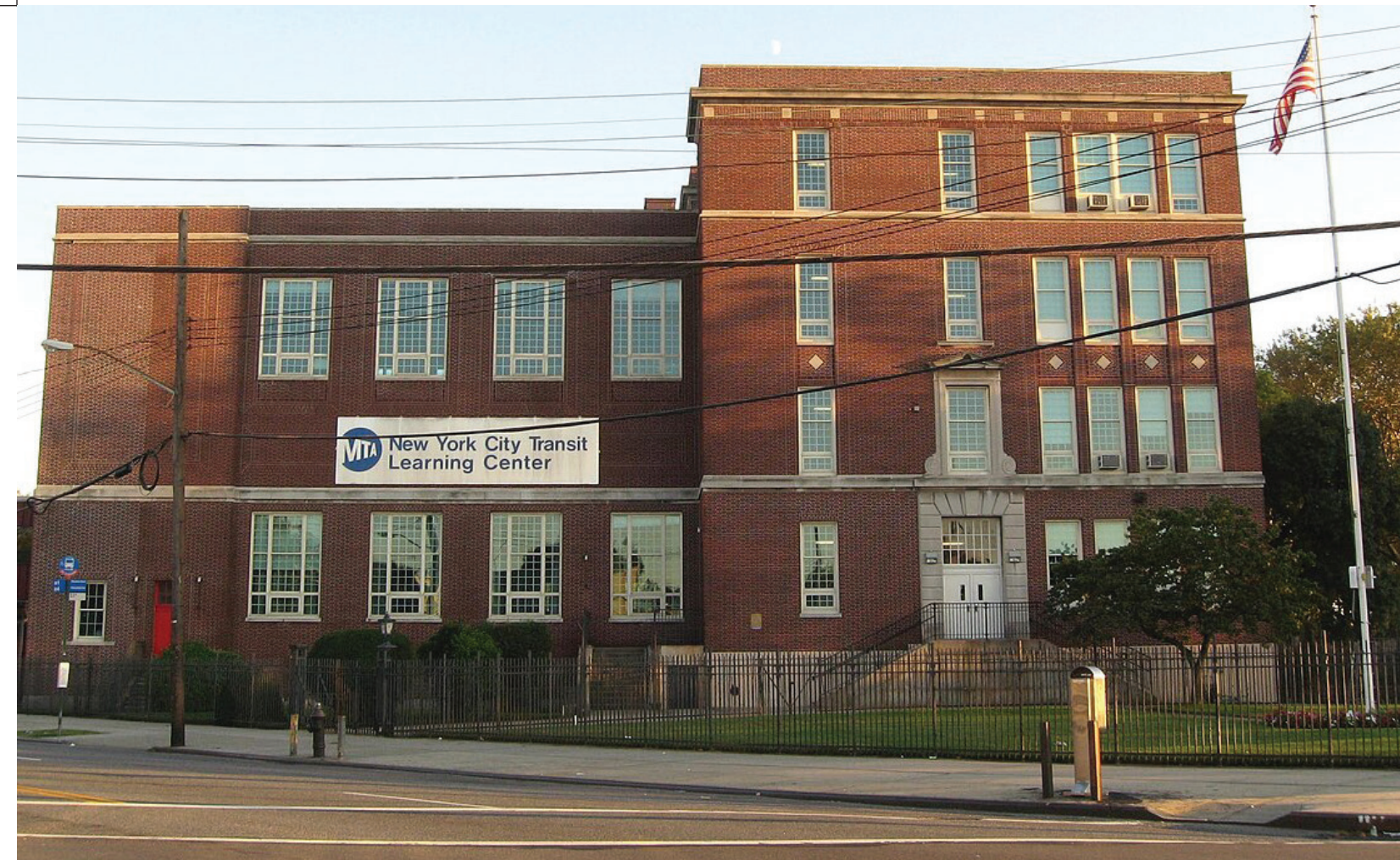
Looking southeast across 86 Street and Avenue U, at New York City Transit Learning Center in Gravesend, Brooklyn
