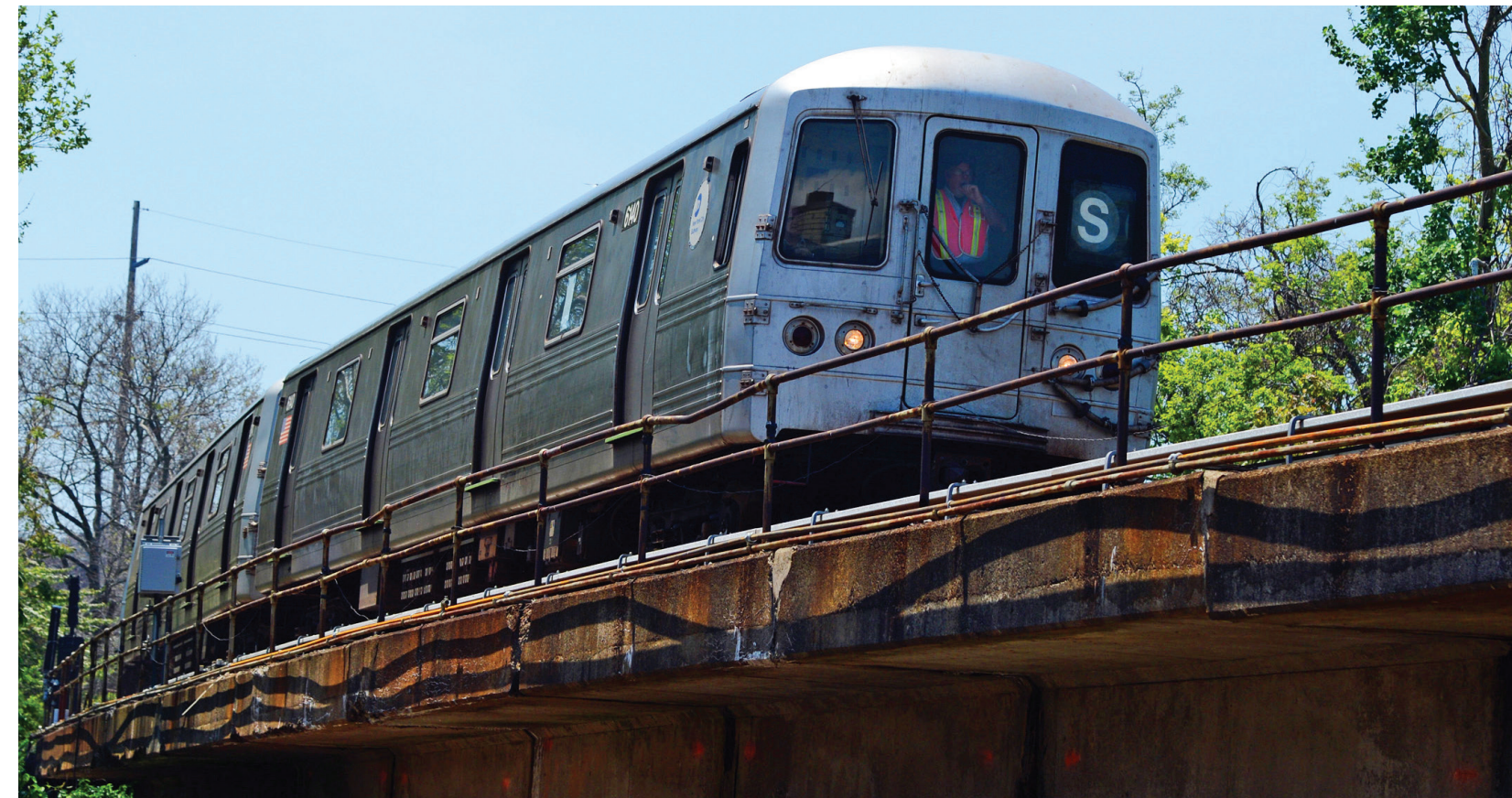
Rockaway Park Shuttle train crossing Hammels Wye, NYCT
