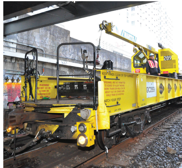
Work train with crane
