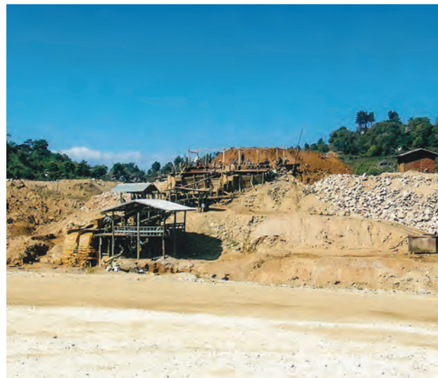
Figure 20: The washing plant at the Lian Shan mine is fully mechanized. Photo by U Tin Hlaing.
