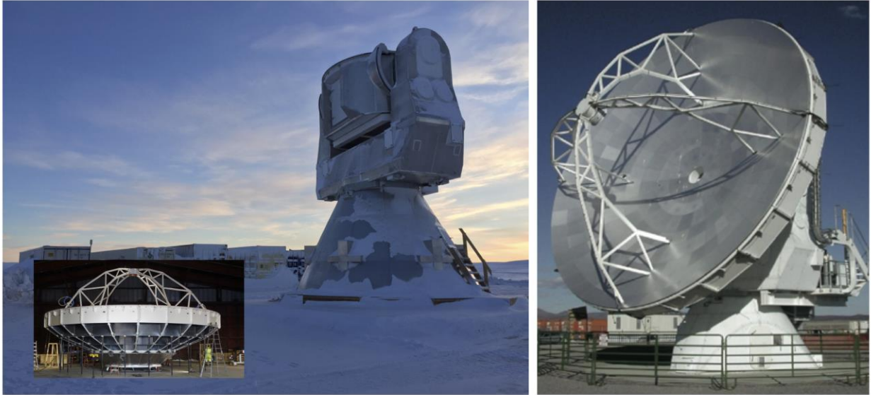
Figure 4.2.1: (Left, and inset): The Greenland telescope antenna under construction at the Thule Air Base (cluster pad 1, and hangar 6). The Alt-Az antenna mount, dish back up structure and quadrapod feed legs are fully assembled, as of August 2016. The antenna construction will be completed in August 2017. (Right): The ALMA prototype antenna at NRAO JVLAsite near Socorro, NM, in 2011.
