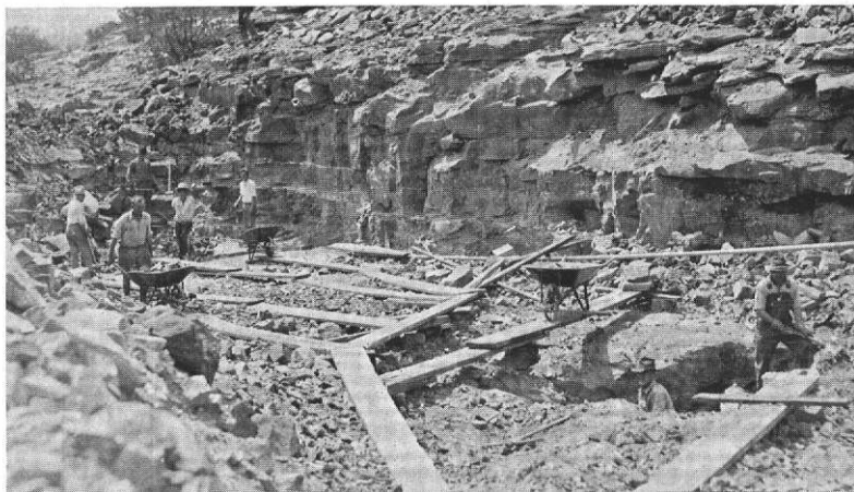
B. Bituminous sand quarry of the New Mexico Construction Co., 10 miles north of Santa Rosa, San Miguel County.
