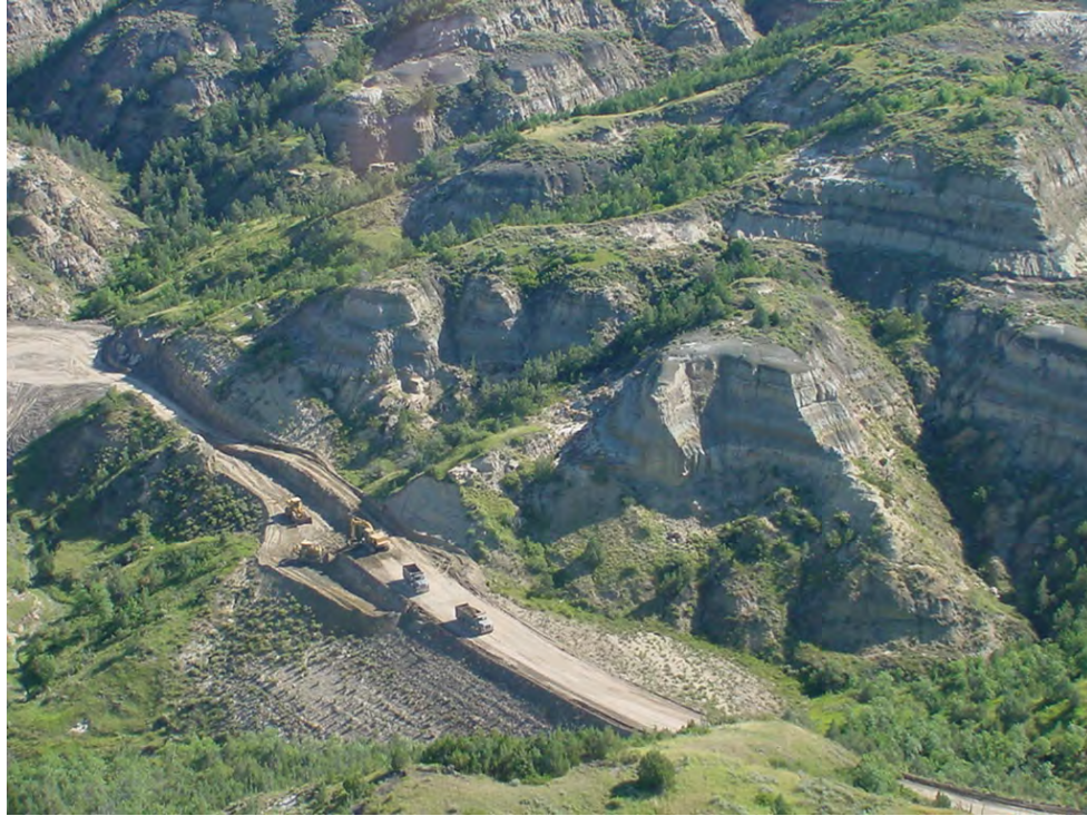
Figure 10. Oil road construction through bighorn habitat near Magpie Creek.
