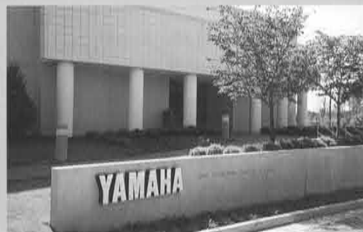
YMMC is a 500,000 square-foot facility located in Newnan, Georgia just south of Atlanta
