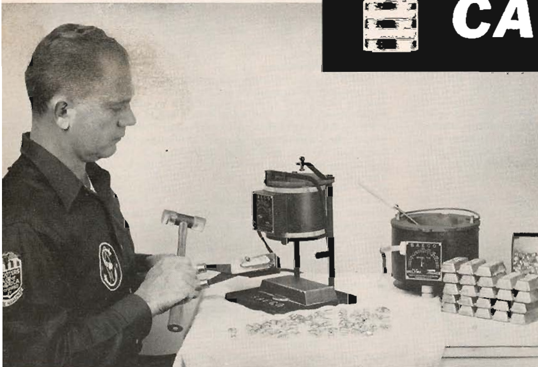
The author uses either the bottom draw thermostat furnace or the Thermo-Utility dip pot, both made by SAECO, depending on the type of mould he wishes to use.
