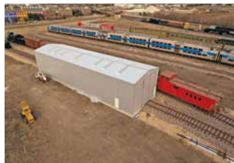
The Museum of the American Railroad has completed its first new building, a 30 x 108 repair shop and earlier in the year laid its last three yard tracks.
