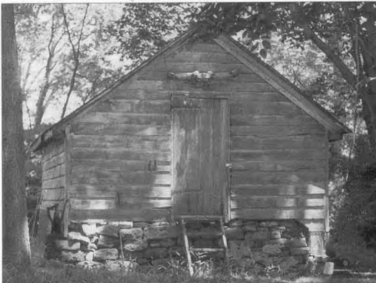
Shed at the Garret Durie House
