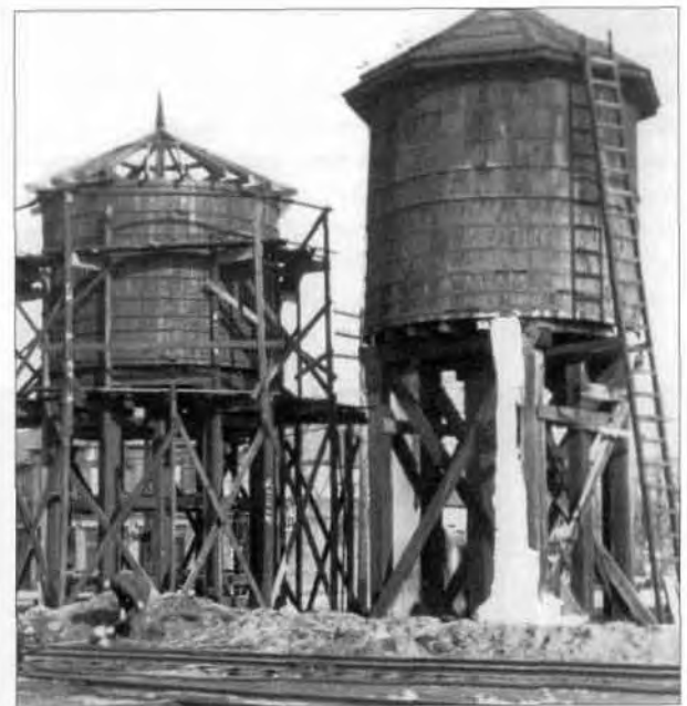
Hillsdale's water tower in the process of going from old to new. The "new" tower was eventually torn down, signifying the end of the era of the steam locomotive.
