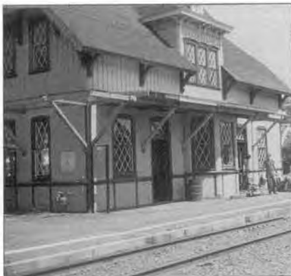
Train Station under Renovation
