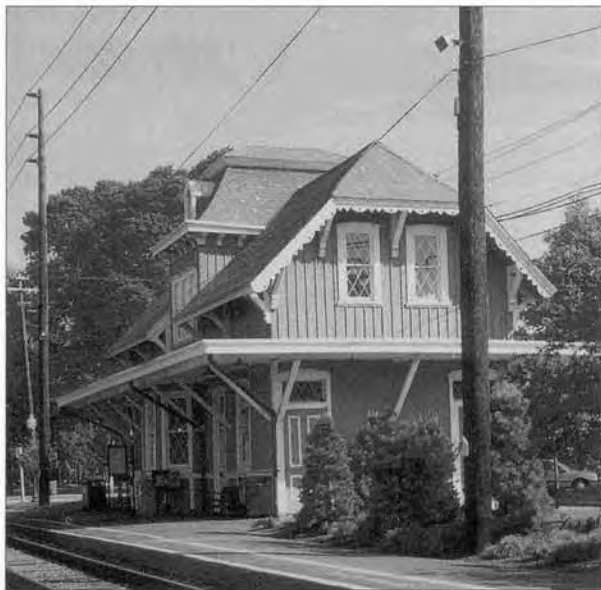
Hillsdale Station today.
