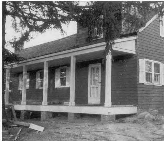
Forshee-Blauvelt-Demarest House - late 1700's, seen here undergoing renovations
