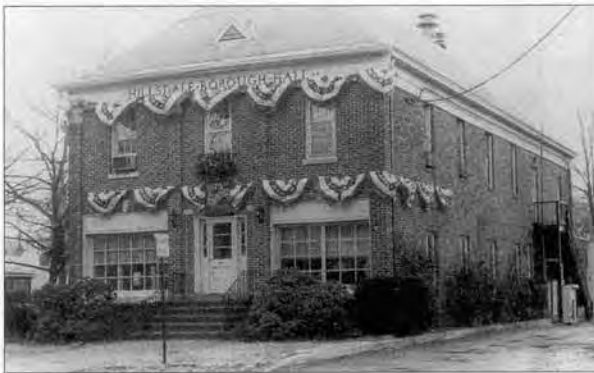
Borough Hall building in 1973 just prior to its demolition.
