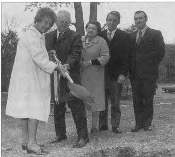
Members of the Board of Trustees at the ground breaking for the addition to the library in 1972.
