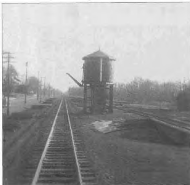
Water tower center with turntable just in front of it. Note second set of train tracks as well.
