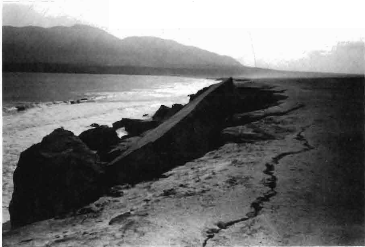
Fig. 1.2.1.- To the west of La Portada, evidence of superficial fracture and gravity sliding along the edge of the seacliff, produced by the July 30, 1995 earthquake.
