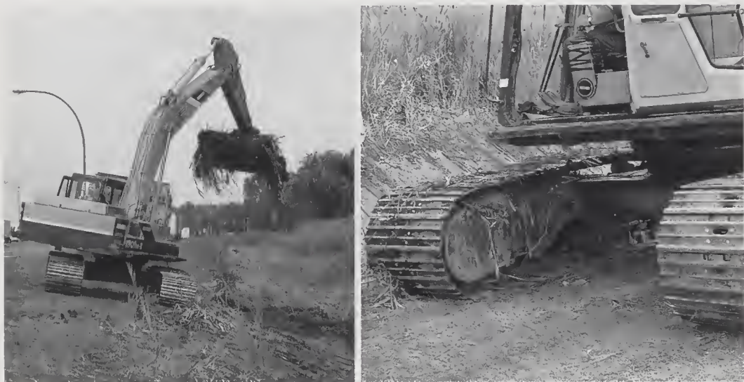
FIGURE 7. An excavator working along a highway in southwestern Quebec, where it is being used to deepen a roadside ditch. The excavated substrate containing rhizomes of Phragmites australis subsp. australis will be transported to a landfill, and rhizomes with shoots can be seen lodged in the tracks. The vehicle will likely introduce rhizomes to the next work site. Photo by P.M. Catling in southwestern Quebec in 2005.
