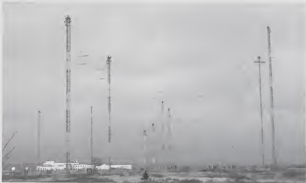
FIGURE 3. Radio Canada International station situated on Coles Island within the Tantramar Marsh near Sackville, New Brunswick. There is a complex matrix of wires/guy lines between the towers. The tallest feature is 131 m. Photo: C. MacKinnon.
