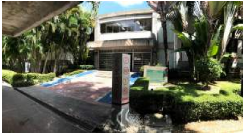
Fig. 1. View of EP Building.
