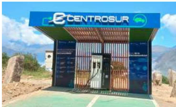
Fig. 11. Charging station - Installation
