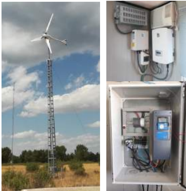
Fig. 1. Wind energy system composed of a Ryse Energy E5, a DC/AC inverter and a DC/DC converter.
