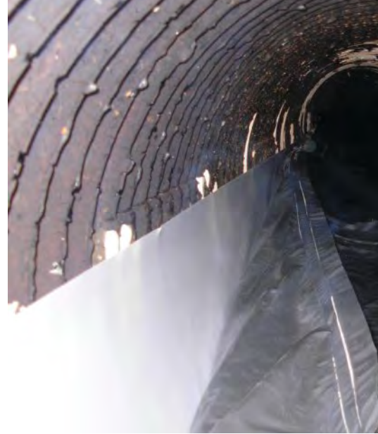
Relining with Blue-Tek ultraviolet curing system
