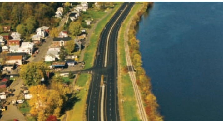
SR 7 in Monroe County, the first ODOT project to include a warranty, was constructed by Shelly & Sands in 1997.
