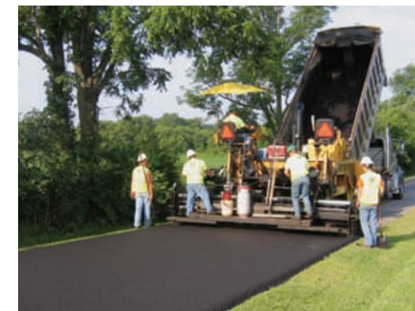
Asphalt 404-LVT proved to be a better value than surface treatments for rehabilitating low volume pavements, first placed in Fayette County in 2009.
