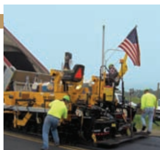
National demonstration of Warm Mix Asphalt technologies on SR 541.
