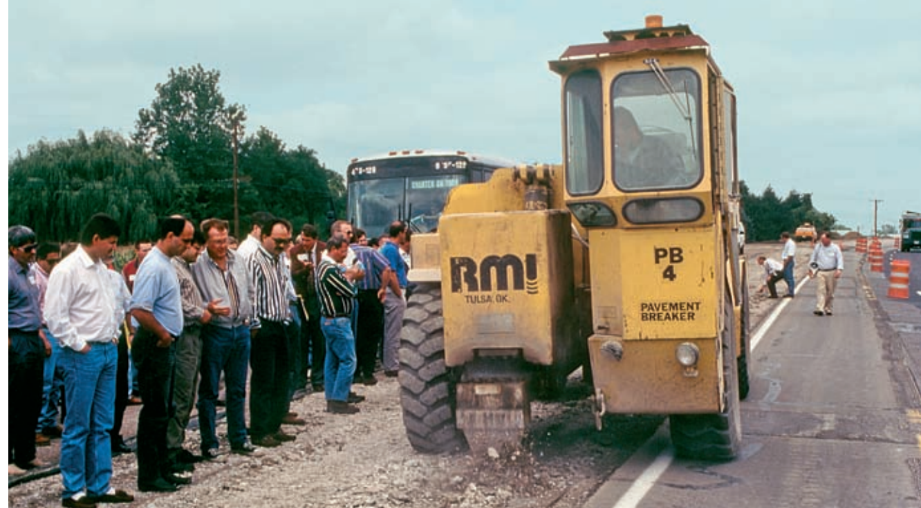
Fractured slab technologies, such as rubblization (above) and break-and-seat (left) helped expedite construction and improve safety and travel through work zones.
