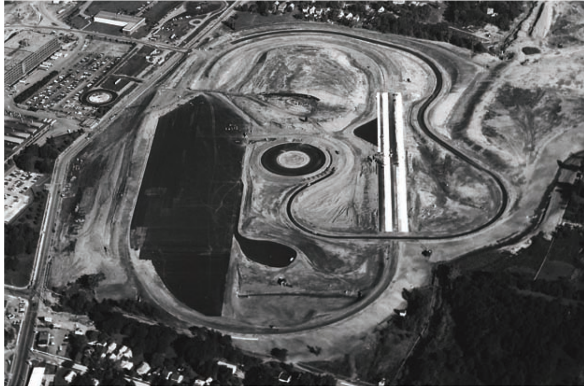
The Goodyear Test Track in Akron, paved by Thomas Asphalt, featured a 60,000 sq. yd. vehicle dynamics area, a main track of about one mile in length, an acceleration area, tethered circle, and a simulated paved area involving special surface finishes.
