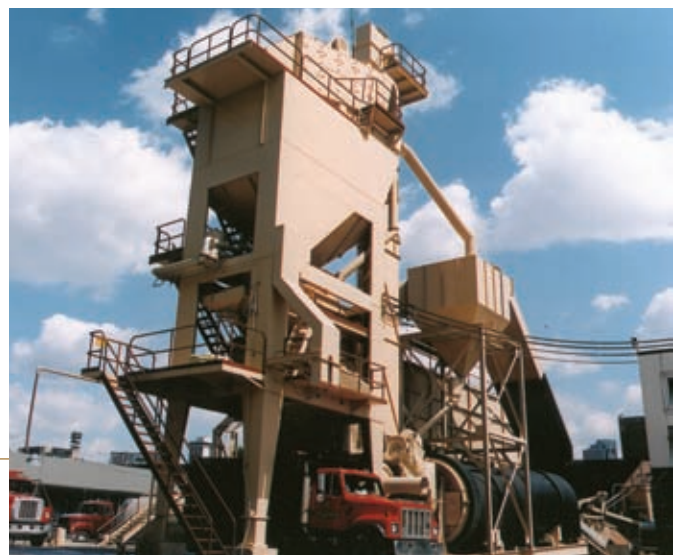
FPO and the Ohio EPA worked toward the standardization of practices among OEPA districts to help streamline operations.
