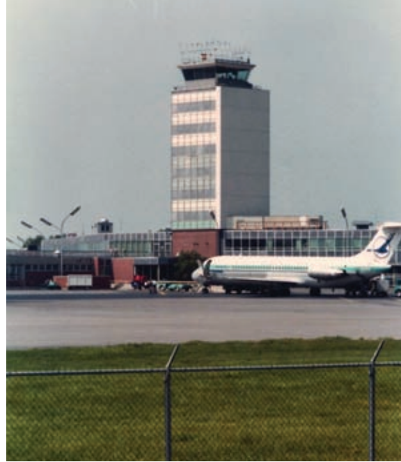
The use of hot-mix asphalt increased in all areas of transportation, including the runways of Port Columbus Airport.
