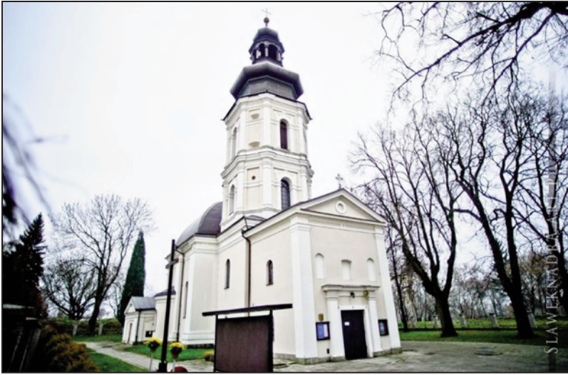
FIGURE 4. Church of St. Nicholas in Zamosc where the Synod was held. Its architects were John Wolf and Yaroshevich who built the new brick church in the Baroque style. In the 1690s the octagonal tower was added. Photo made available under the Creative Commons Attribution-Share Alike 2.5 Generic, 2.0 Generic and 1.0 Generic license, by Wikimedia Commons user MaKa-commonswiki. https://commons.wikimedia.org/wiki/File:Mikolaja8.JPG
