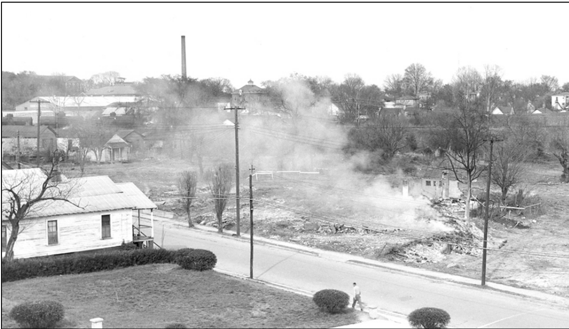
Looking northeast. Courtesy Raleigh Housing Authority.
