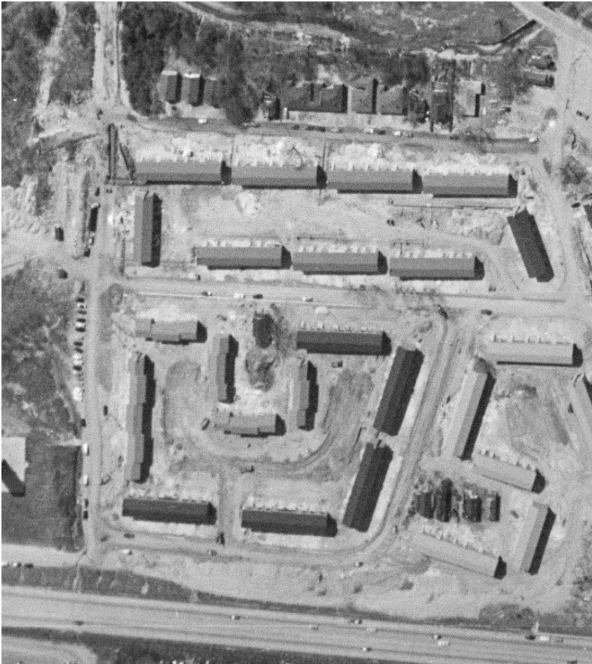
Aerial photo of construction, 1959. USDA Historical Aerial Photo.
