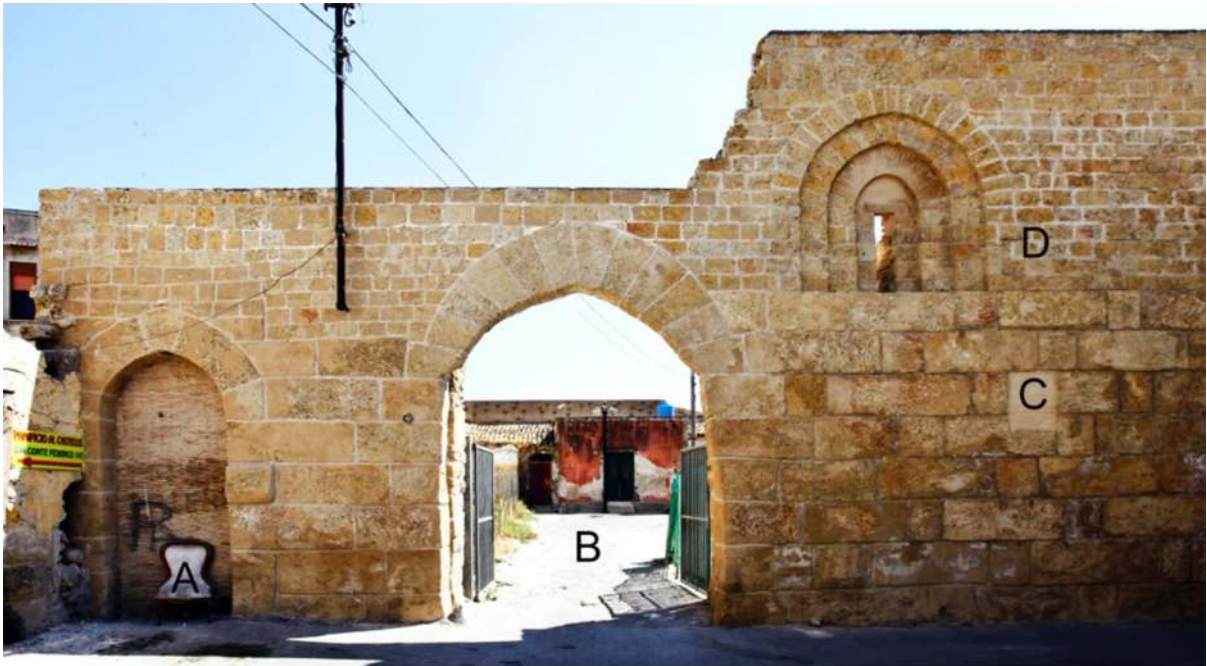
Figure 7 – Mareдолce Palace: a) door from the Islamic period; b) door of the Modern period; c) northern side of the Islamic building; d) upper part of the building in the Norman period (photo from the Soprintendenza BBCCAA of Palermo)
