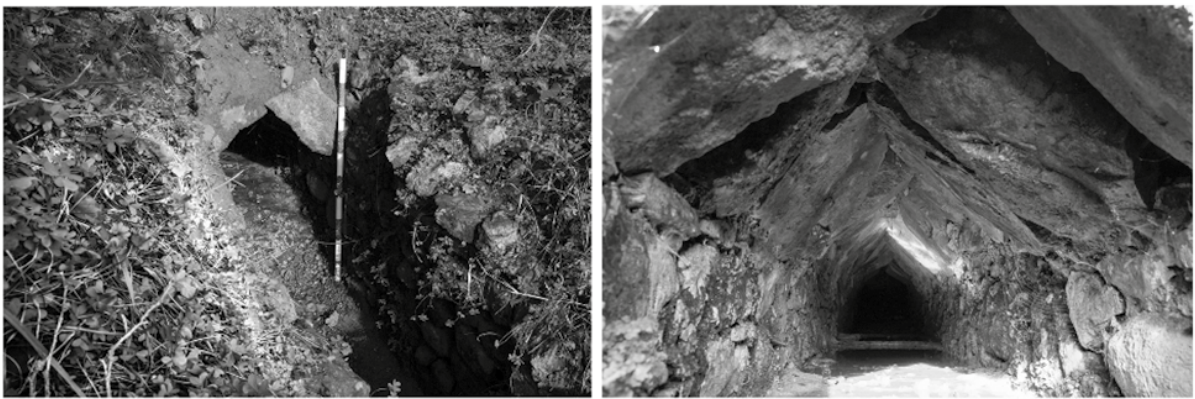
Figure 6 – Exterior and interior of a drainage gallery in Contrada Pietralia
