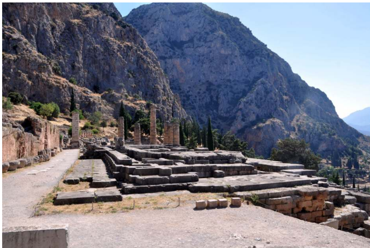
Figure 8: Temple of Apollo. Distortion of the euthynteria .
