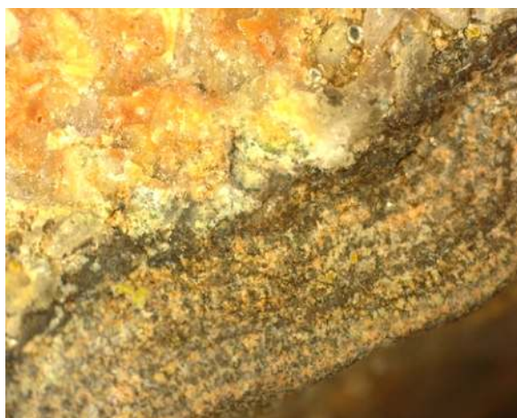
Figure 11: Solunt. Digital microscope details of the laminations of the SOL 18/19 sample at the architectural block of the 'Edificio sacro a due navate' (photo: V. Ollivier).
