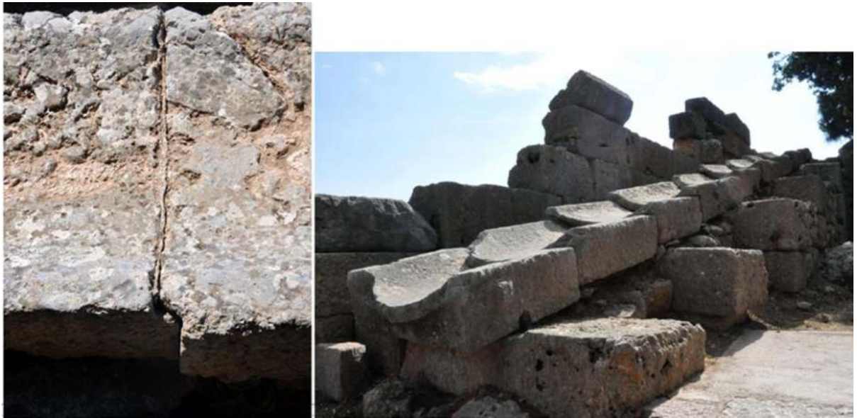
Figure 10: West Stoa: detail of the north gutter sealed with lead; east part of the north gutter.
