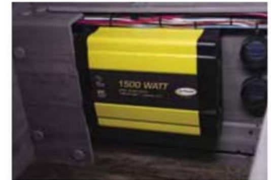
Optional 1500w inverter allows your battery-based system to run conventional appliances by inverting 12V DC to create 120V AC output. - N/A 2465
