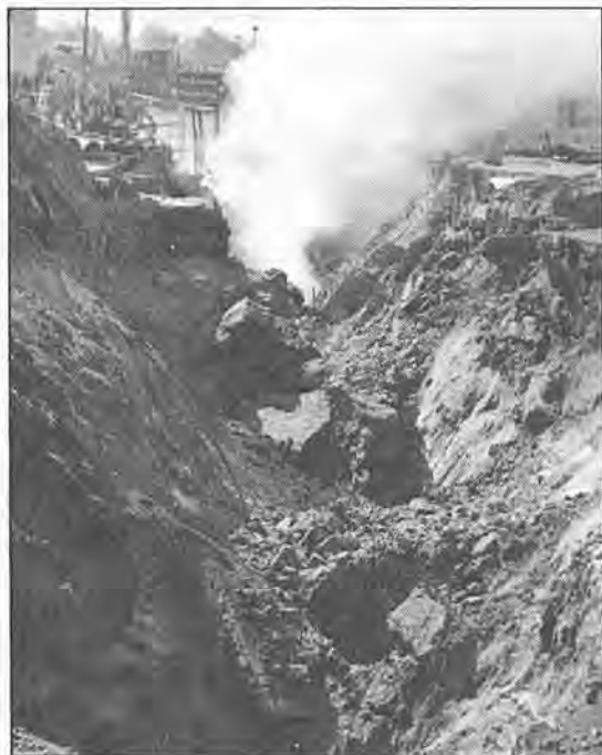
Within 10 feet of the quieted freeway, the tunnel caved in. At the end of the elongated fissure in the earth, smoke spewed out.
