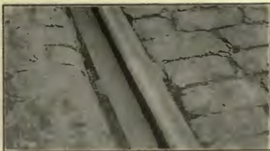
A Thermit Rail Weld made over five years ago in Grand Street, Jersey City, N. J., and still as good as new.
