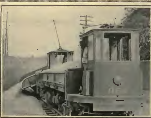
"Differential Two-Car Train. Trailer dumping load clear of trench."
