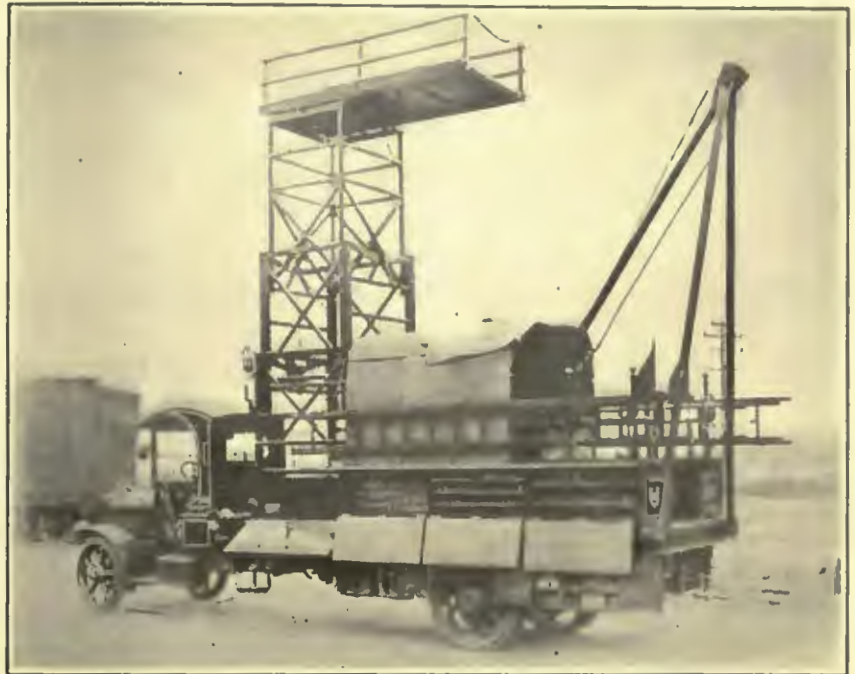
A White combination tower and line construction truck in the service of the United Electric Railways, Baltimore
