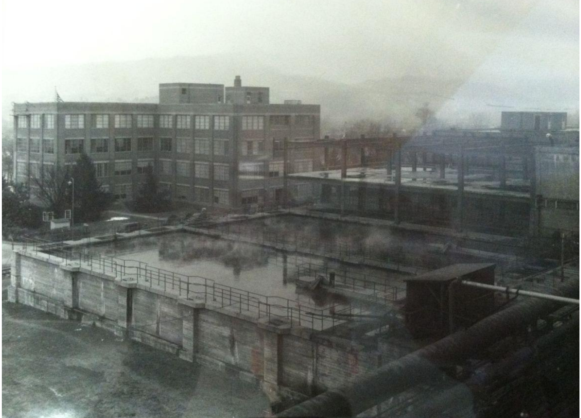
February 1948 B-54 filtered water basins
