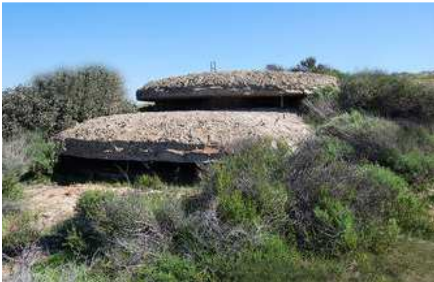
Typical WWII San Diego Pillbox Similar to the One at Bird Rock
