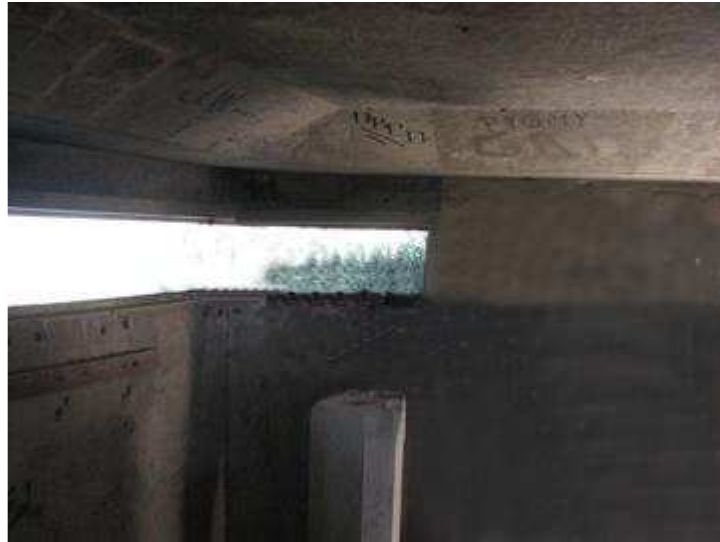
Typical Pillbox Interior. Note cement base for machine gun
