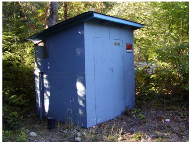
Minerva Well Control Building
