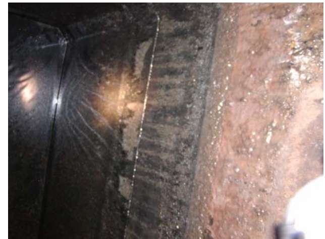
Potlatch State Park – RV Dump Septic Tank
