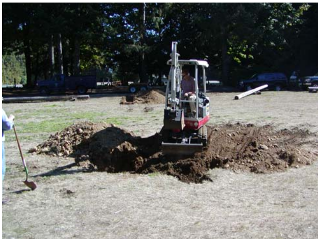
Minerva Beach - Drainfield Test Pit
