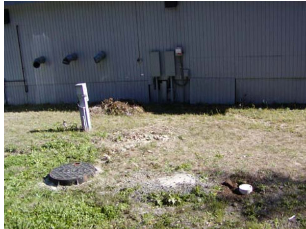
Minerva Beach - Laundromat and Pump Station Controls
