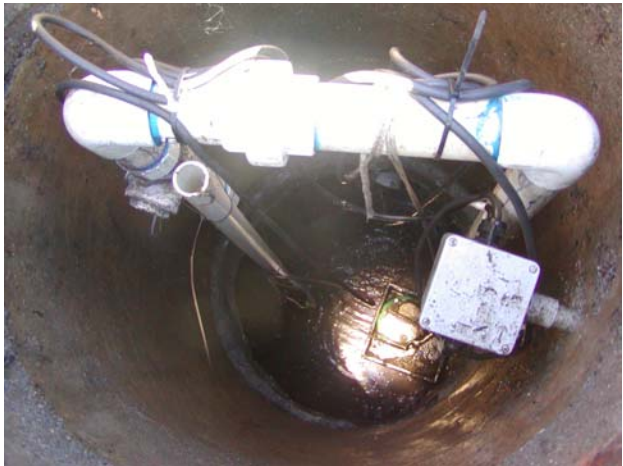
Minerva Beach - Laundromat and Pump Station
