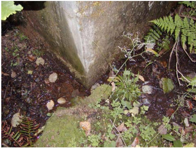
Minerva Water Storage Tank
