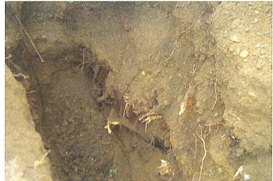
PHOTOGRAPH OF TEST PIT
