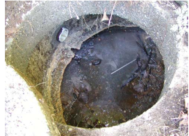
Minerva Beach - Drainfield Manhole
