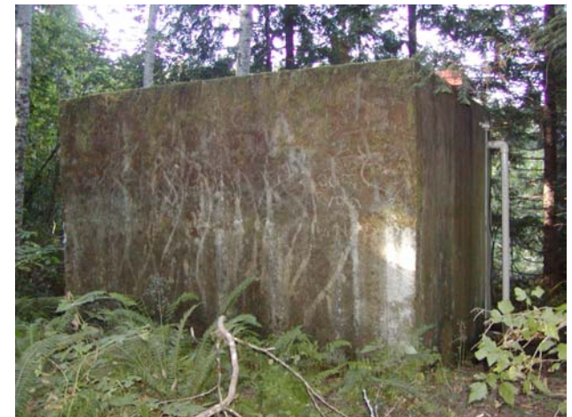
Minerva Water Storage Tank
