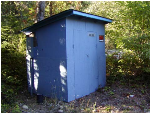
Minerva Well Control Building
